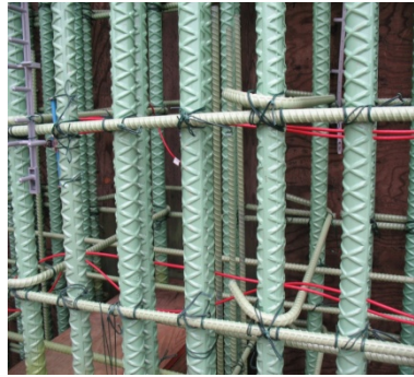
Fig A.3.5.3: Gauge leads being run to PVC transfer pipe.
