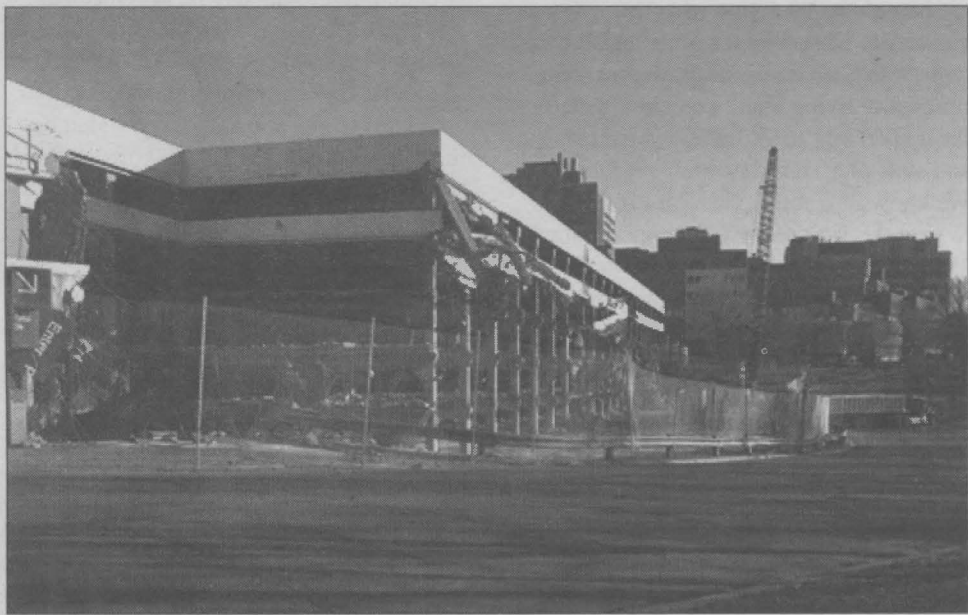
Demolition of the East River Road parking ramp axed 1,700 parking spots. Demolition began in October...
