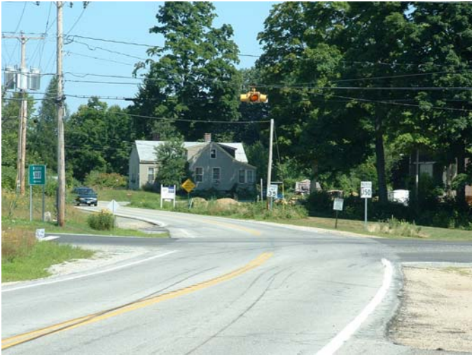
FIGURE 4-11 Horizontal Curve in NH 150 Alignment
