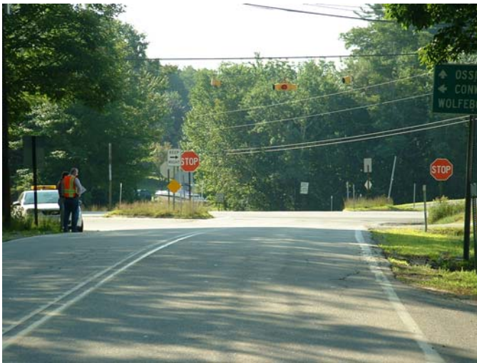
FIGURE 4-6 Dual Stop Signs on West Approach
