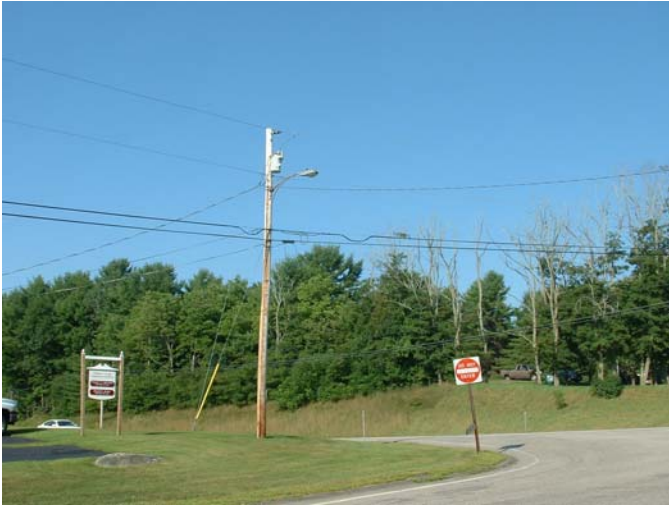
FIGURE 4-5 Intersection Lighting in Southeast Intersection Quadrant
