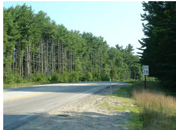
FIGURE 4-7 Vertical Crest and Horizontal Curve North of Intersection Viewed from West (left photo) and East (right photo) Approaches
