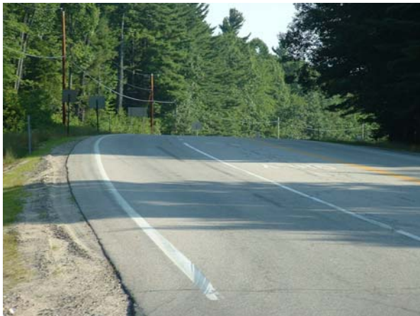
FIGURE 4-7 Vertical Crest and Horizontal Curve North of Intersection Viewed from West (left photo) and East (right photo) Approaches
