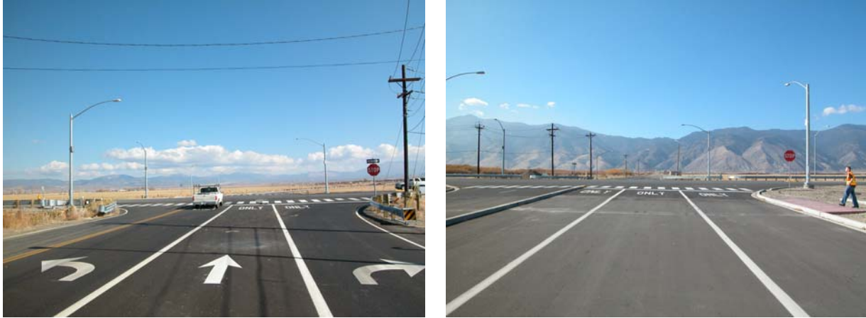
FIGURE 4-6 Approach Design for the West (left photo) and East (right photo) Approaches
