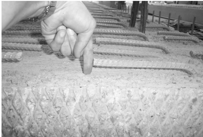
Figure 5.19: Clear spacing under rebar hooks in Center City Bridge precast section
