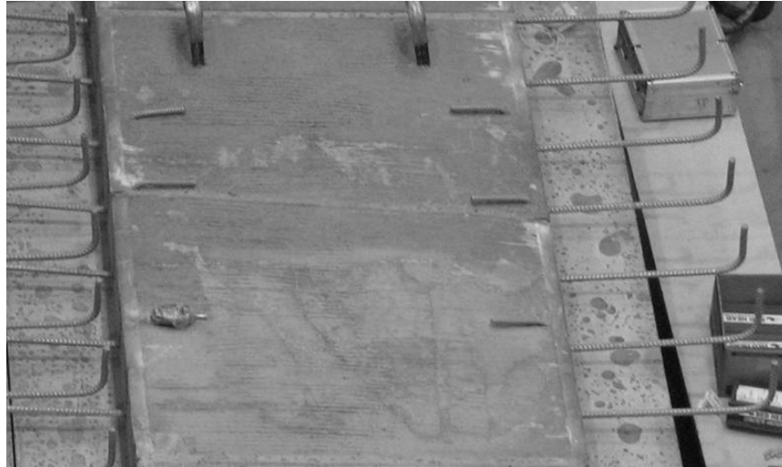
Figure 5.15: Unintentional roughness of flange surface due to shallow air voids
