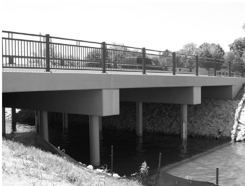
Figure 3.1: Photograph of the Center City Bridge
