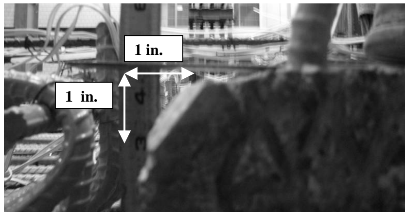
Figure 5.17: Modified 1 in. by 1 in. chamfer in north beams
