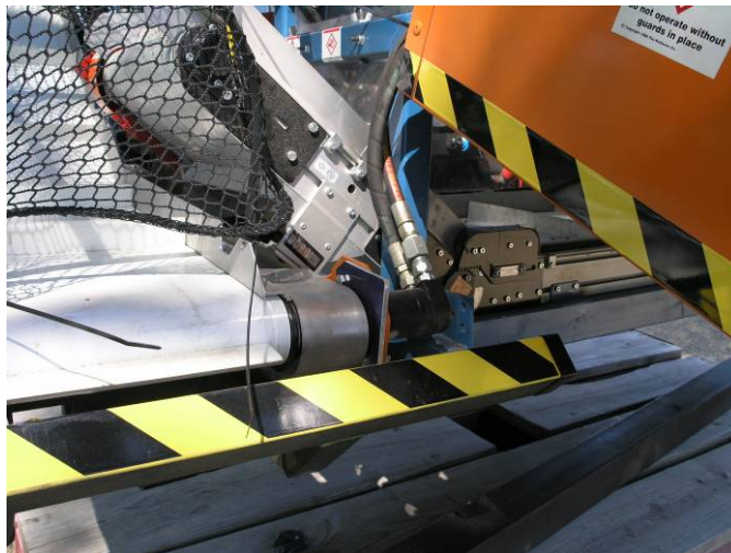
Figure 71: Conveyor Drive Motor
