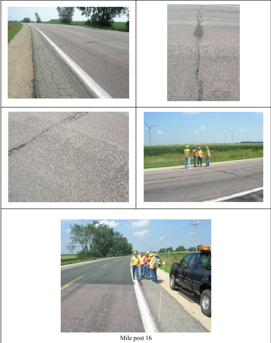
Figure C.5. TH 56 sections with surface treatment applied in 2000 (built in 1995), mile 15 to 16 (Note change in aggregate at mile post 16 from New Ulm quartzite to Dresser trap rock)
