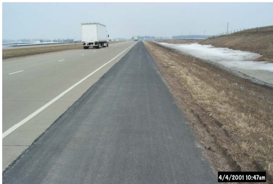
Figure B.2. Almost 100% loss of the seal coat aggregate after the first winter.
