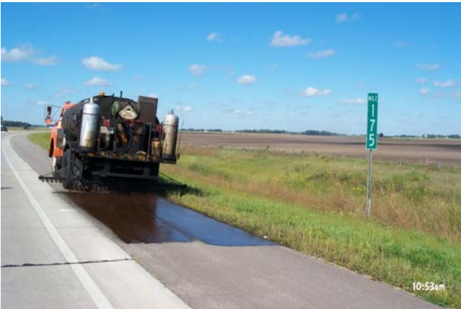
Figure B.7. Starting to apply fog seal
