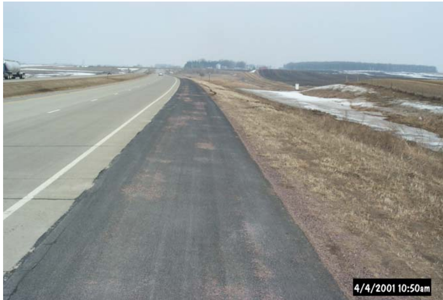
Figure B.4. Shoulder seal coat I-35, R.P. 15-16
