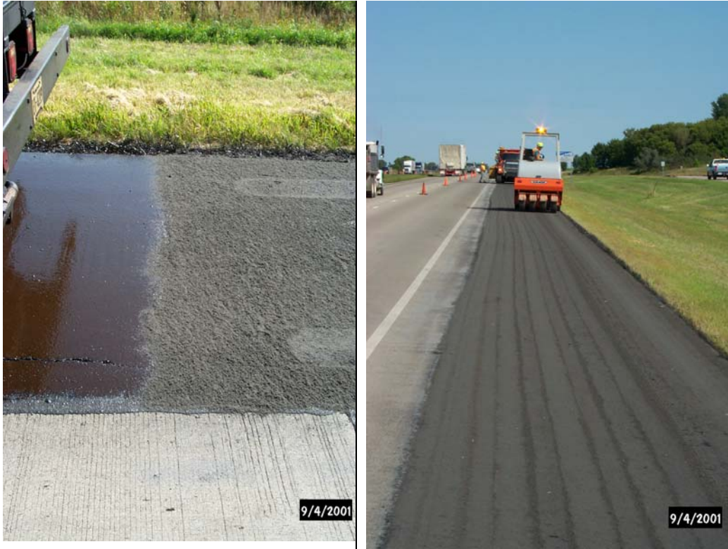
Figure B.5. Shoulder seal coat I-35, R.P. 16-17
