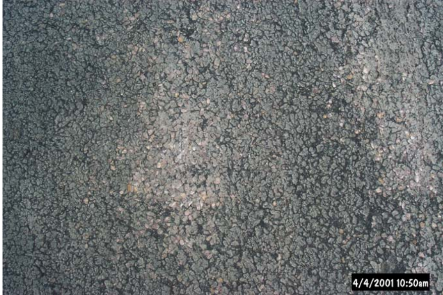
Figure B.3. Close up of shoulder seal coat I-35
