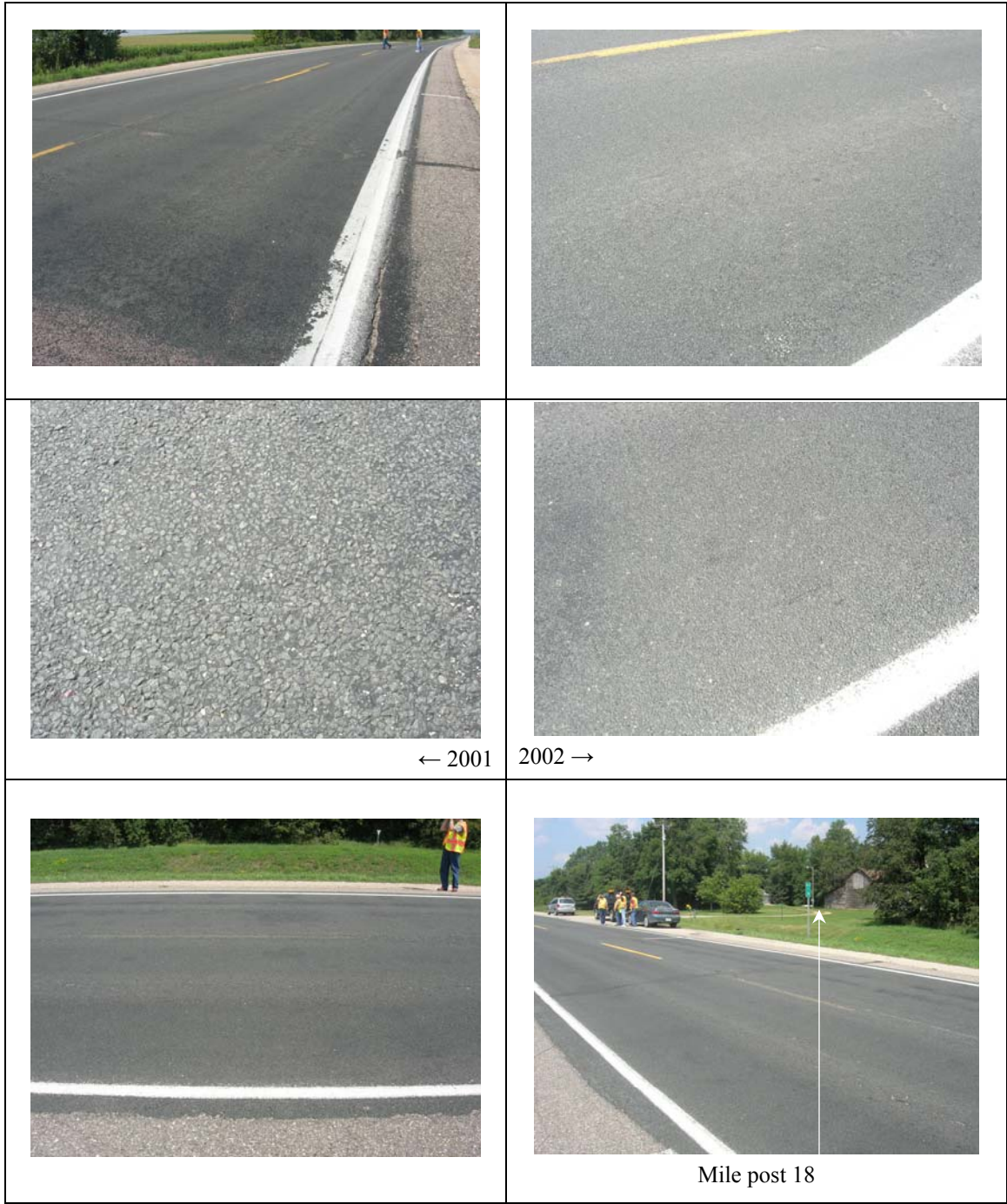
Figure C.6. TH 56 sections with surface treatment applied in 2001 and 2002 (built in 1995), mile 16 to 17 and 17 to 18, respectively
