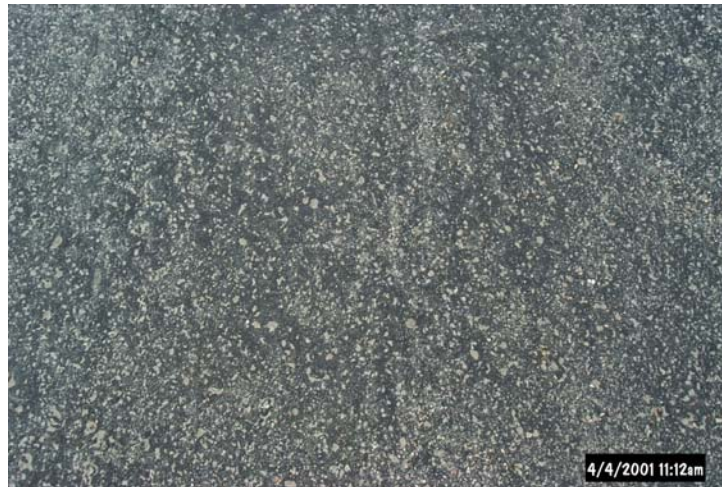
Figure B.10. Close up of fog seal on I-90 after one winter.
