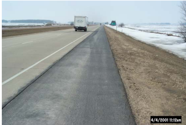
Figure B.9. Fog seal after one winter I-90.
