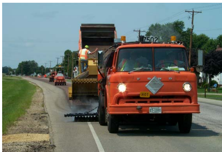
Figure B.1. Applying a Seal Coat to a 1 year old section of TH 56, at R.P. 14 (to 15).
