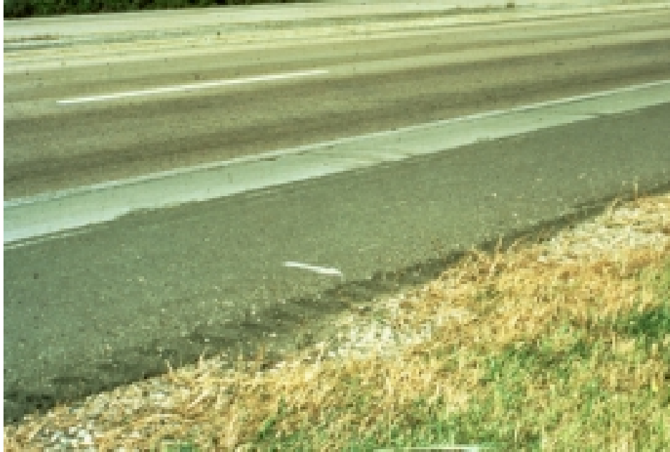
Figure 6.6. Painted arrow as a reference marker (Baumgardner, 2002).
