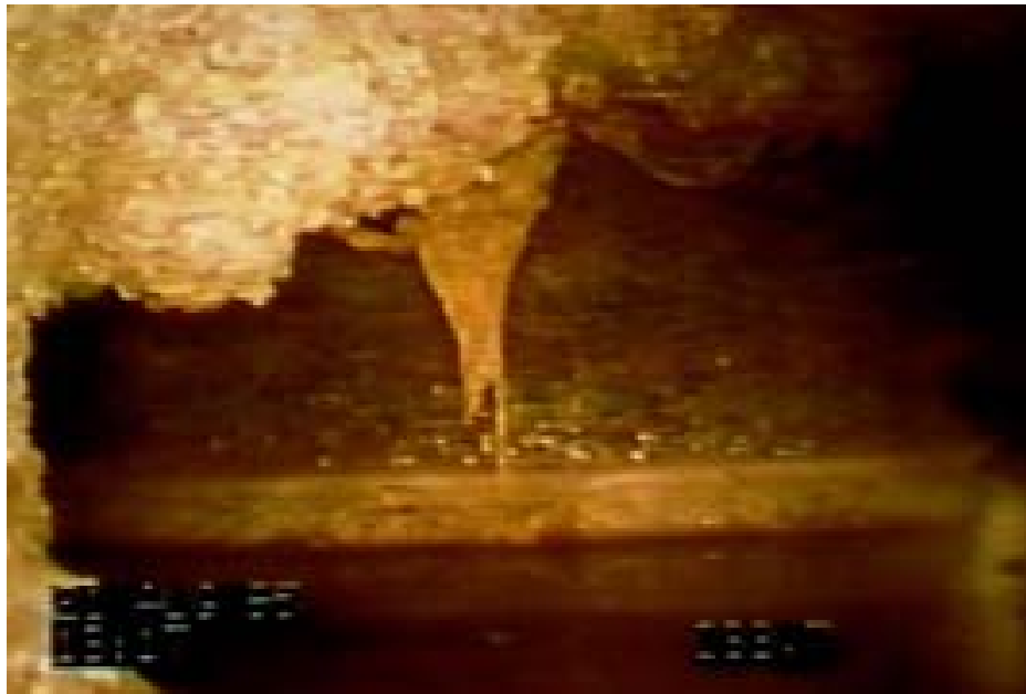
Figure 6.9. Video camera approaching edgedrain (Baumgardner, 2002).
