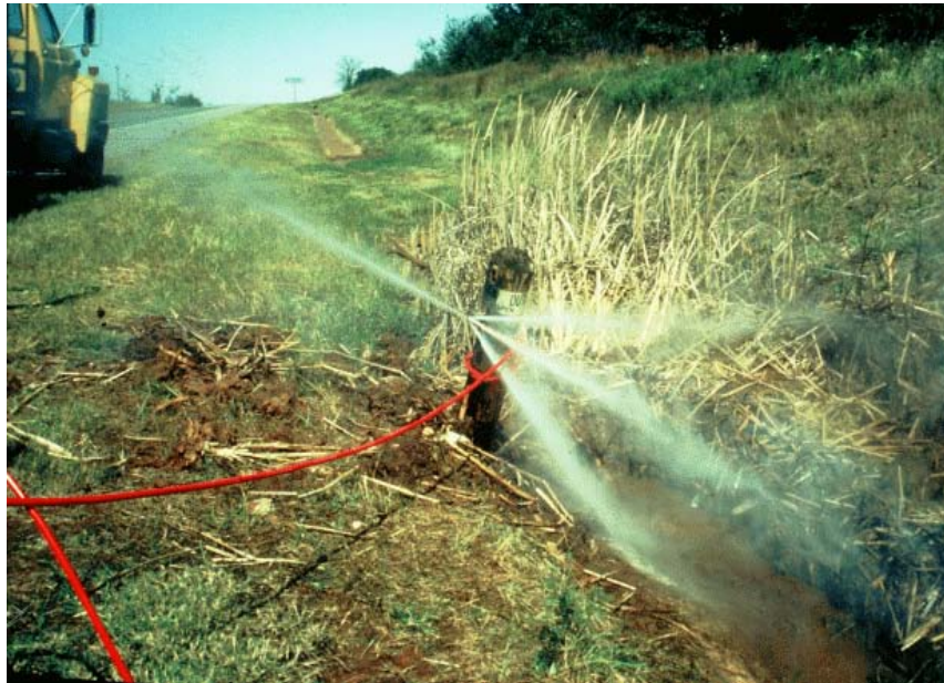
Figure 6.10. Pipe flushing unit (Baumgardner, 2002).
