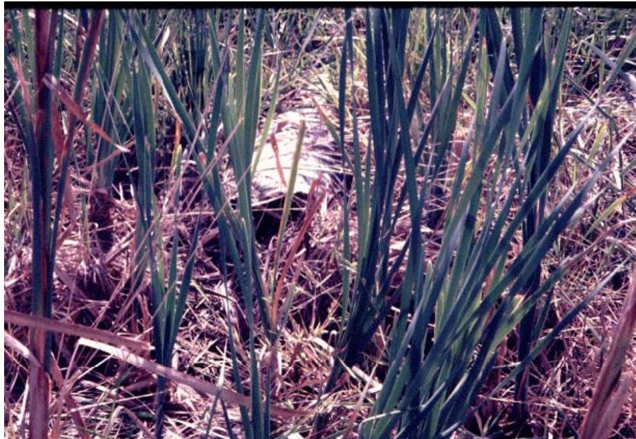
Figure 6.5. Hidden outlet pipe (Baumgardner, 2002).
