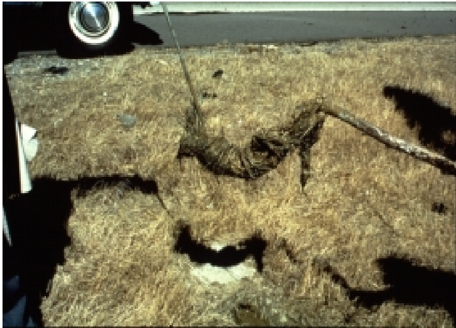
Figure 6.1. Vegetative material removed from an edgedrain system (Baumgardner, 2002).
