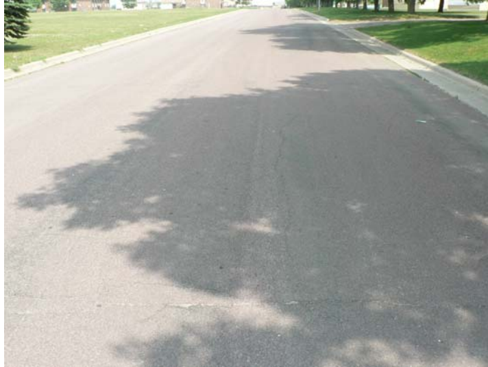
Figure 8.10 View of pavement of Cecillee Street looking east of the intersection with Spring Avenue, showing the presence of some longitudinal and transverse cracks
