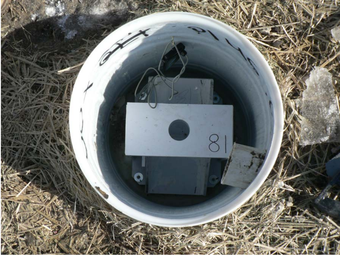
Figure A.4 Levelled tipping bucket ready for connection to the drain outlet from the pavement
