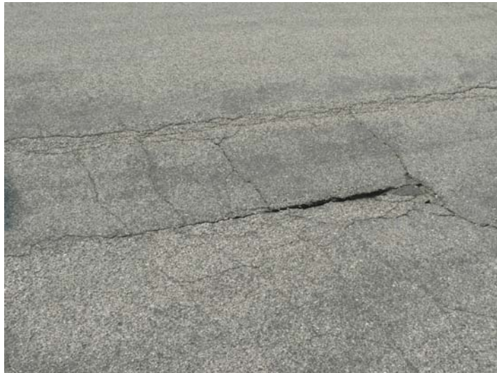
Figure 8.5 Closeup view of cracking on Pleasant Street
