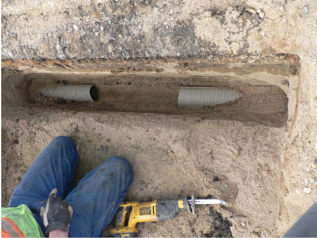
Figure 7.5 Edgeline with tile sample removed
