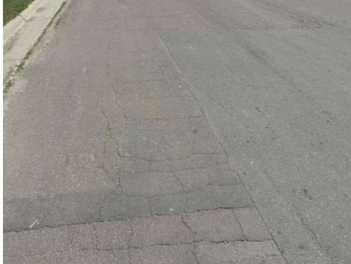
Figure 8.8 View of pavement of N. Spring Avenue, looking south of the intersection with Cecillee Street, showing the cracking pattern in the street
