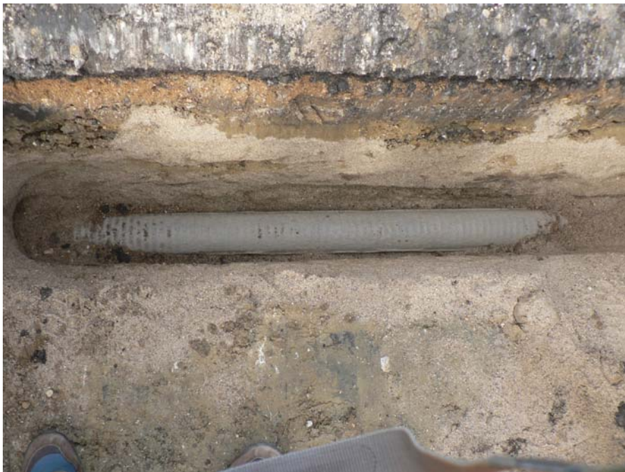
Figure 7.4 Exposed edgedrain at the bottom of the edgedrain trench
