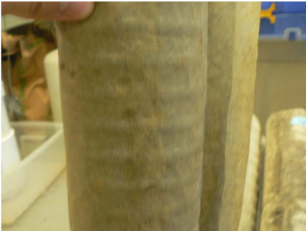
Figure 7.7 The geofabric of the edgedrain at site A on CR 32
