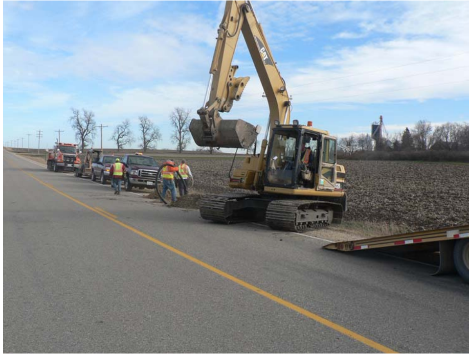
Figure 7.1 Illustration of the tracked backhoe machine used to excavate through the unpaved shoulder to access the edg drain tile on Nobles County CR 32 and CR 35
