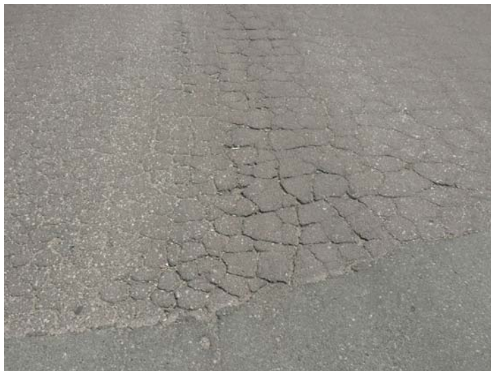
Figure 8.9 Cracking pattern in pavement on N. Spring Ave
