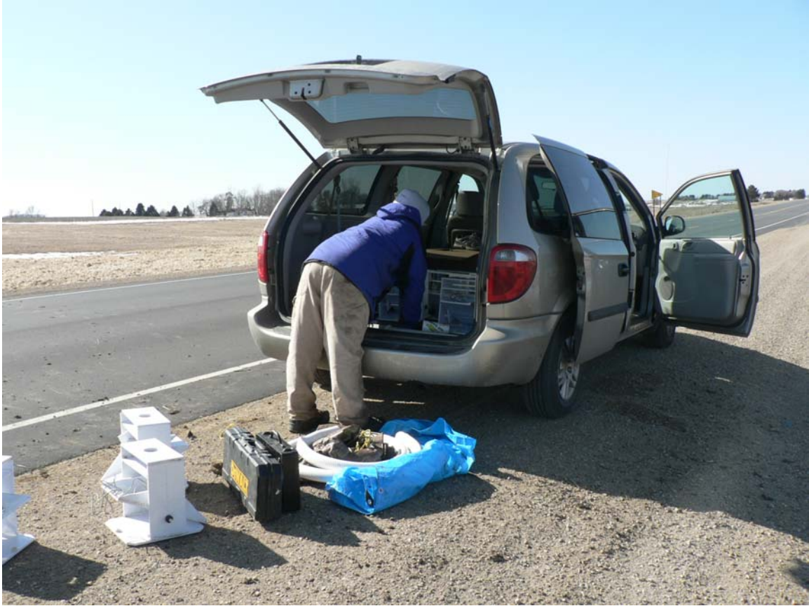
Figure A.2 Preparing materials for installation at a site
