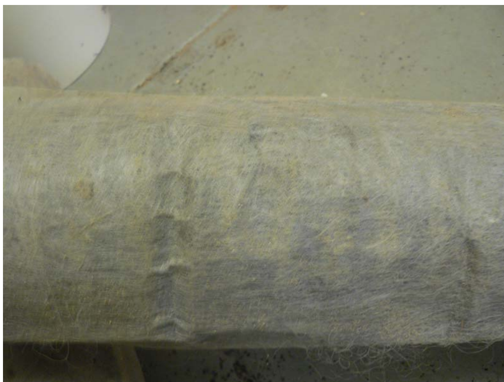
Figure 7.17 The geofabric of the edgedrain at site C on CR 35
