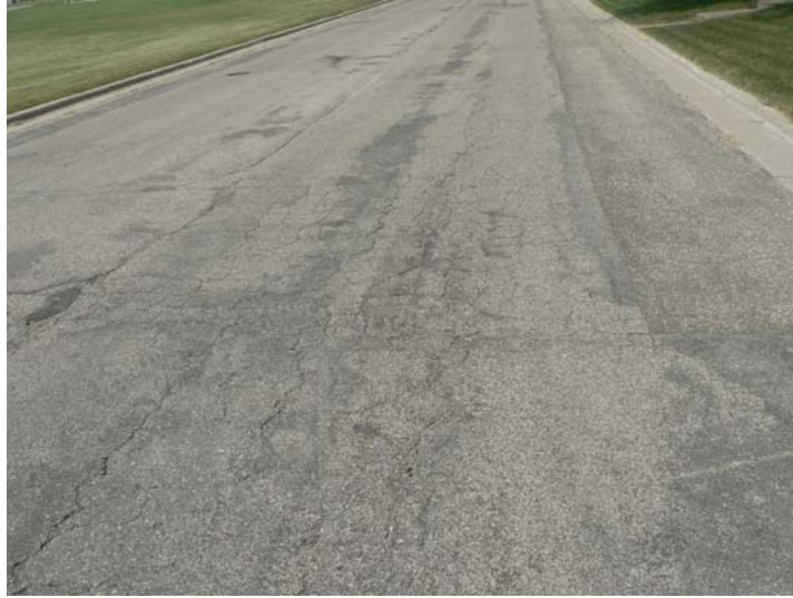
Figure 8.4 View of pavement of Pleasant Street showing the cracking pattern in the street
