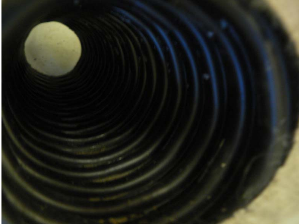
Figure 7.14 The interior of the drain tile at site A of CR 35. There are some deposits on the interior of the drain, but it is quite clean overall
