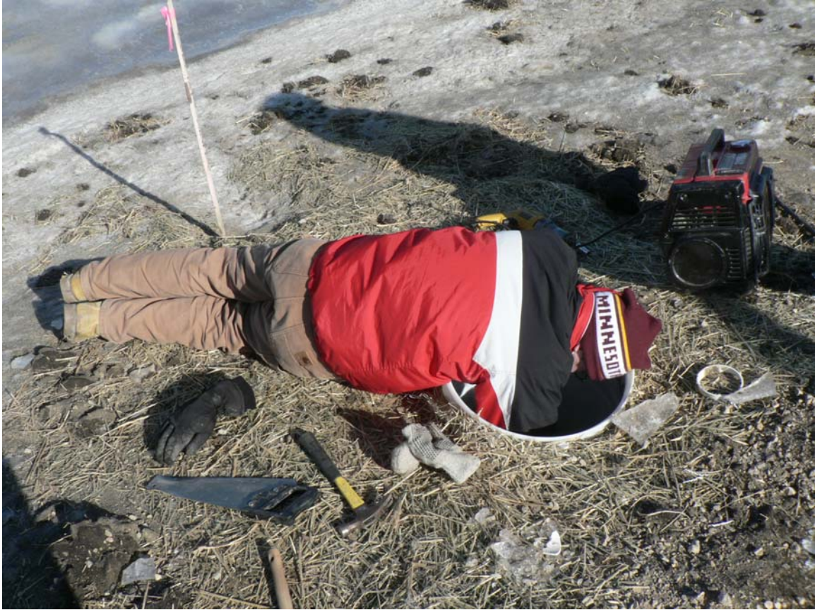
Figure A.3 Preparing the tipping bucket housing and placement of tipping bucket into the housing. Preparation of the tipping bucket in the housing includes the leveling of the tipping bucket
