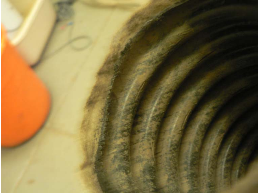
Figure 7.12 The interior of the drain tile at site C of CR 32. Note the deposits
