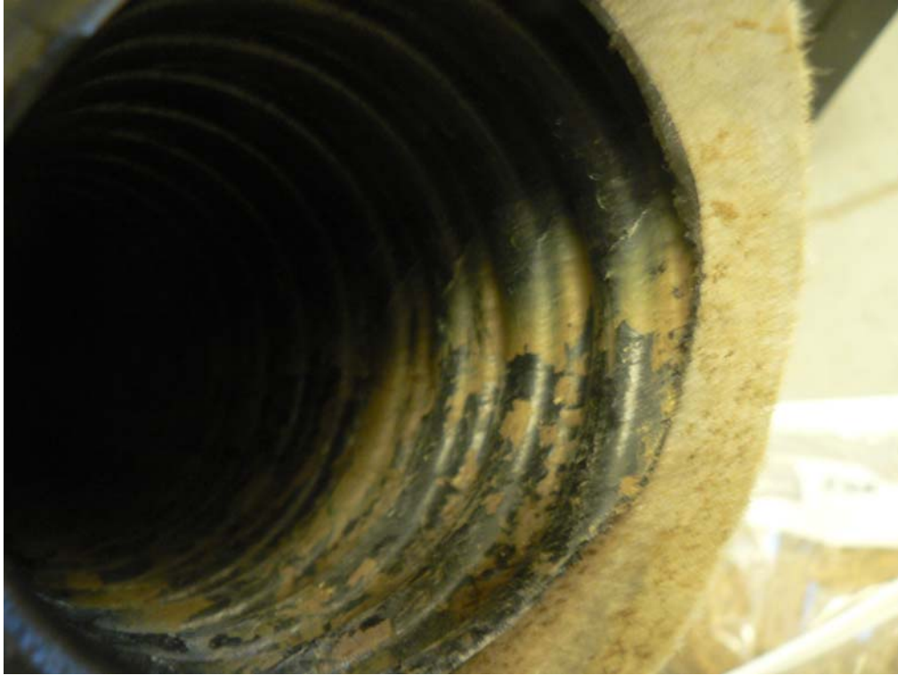
Figure 7.8 The interior of the drain tile at site A of CR 32. Note the deposits on the interior
