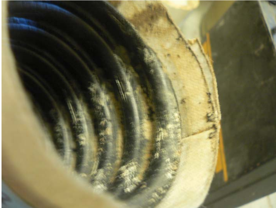
Figure 7.10 The interior of the drain tile at site B of CR 32. Note the deposits
