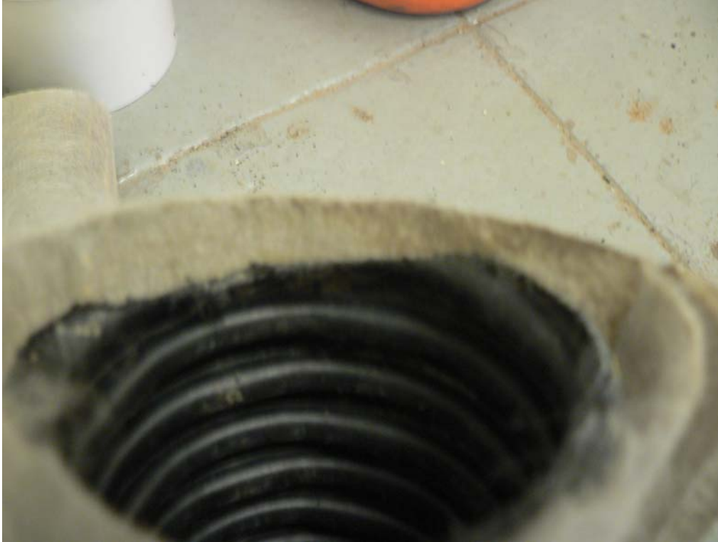
Figure 7.18 The interior of the drain tile at site C of CR 35. Note the deposits
