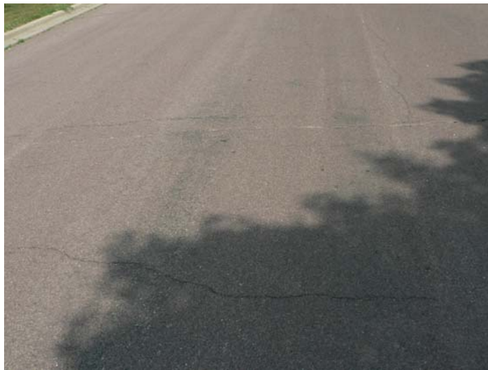
Figure 8.11 View of pavement of Cecillee Street looking west of the intersection with Spring Avenue, showing the cracking pattern in the street
