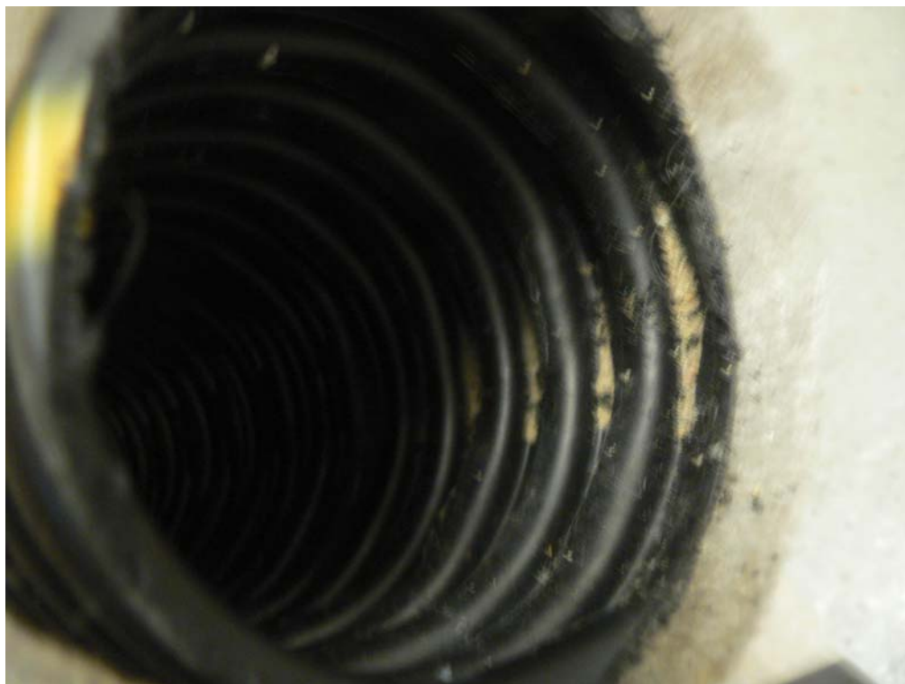
Figure 7.16 The interior of the drain tile at site B of CR 35. Note the deposits
