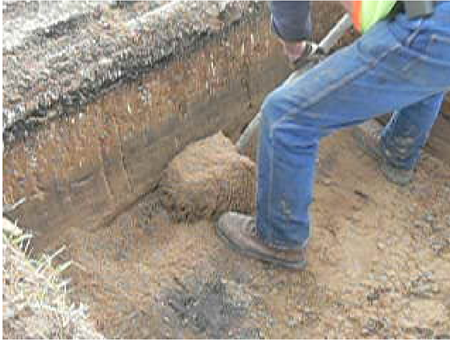
Figure 7.3 Exposing the edgedrain by shoveling out the trench sand
