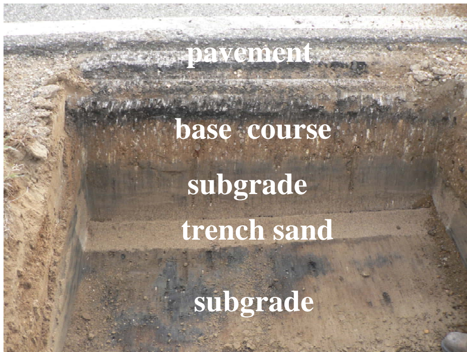
Figure 7.2 Illustration showing the excavated pit down to the level just above the edg drain elevation
