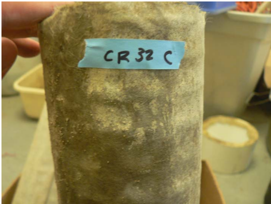
Figure 7.11 The geofabric of the edgedrain at site C on CR 32. Appears to be significant deposits on the fabric material
