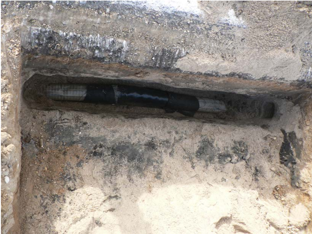
Figure 7.6 The edgeline with the splice in place
