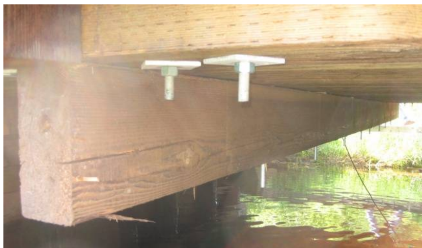
Figure 3.16. Spreader beam mounted below the bridge deck.
