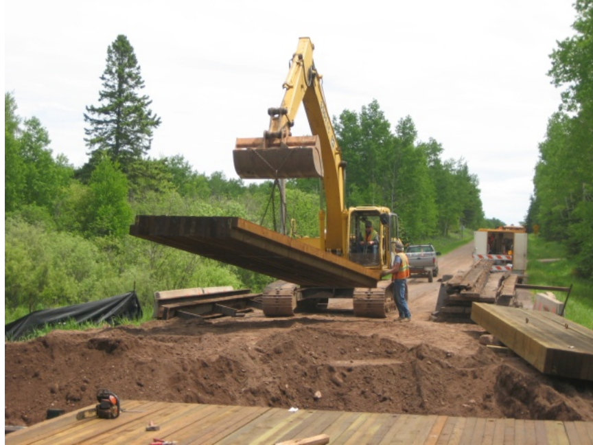
Figure 3.11. Wood sections were set into place using an excavator.
