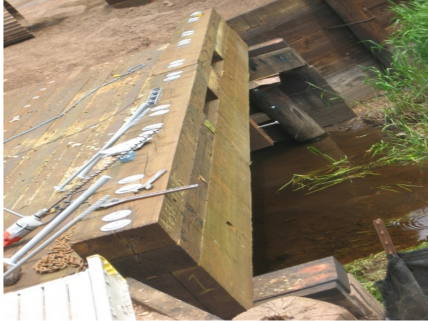
Figure 3.23. Downstream curb completely installed.
