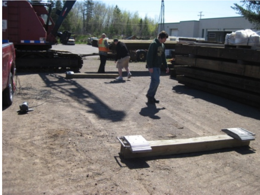
Figure 3.3. Scales were placed on each corner of two beams. The sections were then set on the scales using a crane to get a weight estimate.
