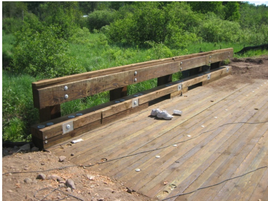
Figure 3.18. Guard rail installed on bridge deck.
