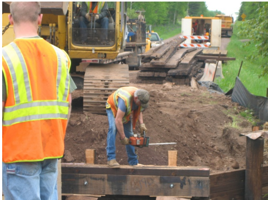
Figure 3.12. Some stays were trimmed with a chainsaw so sections could fit. Copper naphthenate was used to treat the newly exposed surfaces.
