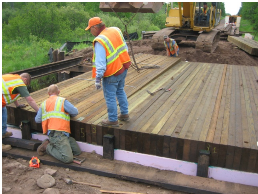
Figure 3.19. The first three sections were set into place and then vibration testing was done.
