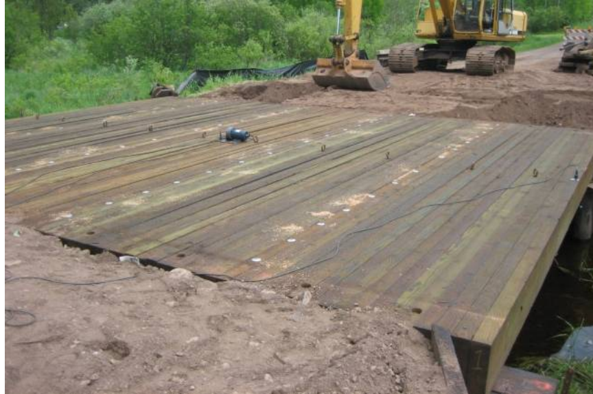
Figure 3.15. Once sections were pinned together and bolted to the pile cap, dirt was back filled.
