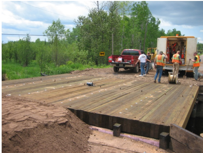
Figure 3.22. Vibration testing conducted with the French River Rd side of the bridge completely back filled and half of the other side of the bridge back filled.
