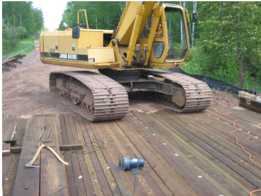
Figure 3.24. Some tests were run with the excavator part way on the bridge deck.
