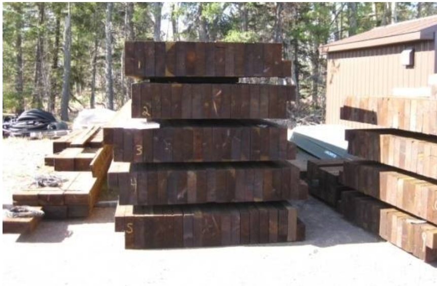
Figure 3.1. Bridge sections to be used as the new superstructure for St. Louis County Bridge 53.
