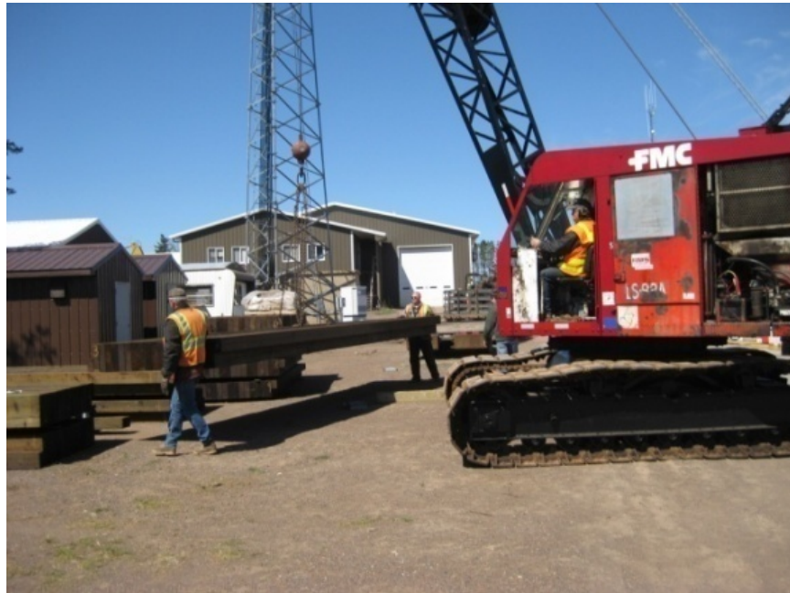
Figure 3.2. A crane was used to transport sections for weighing and vibration testing.
