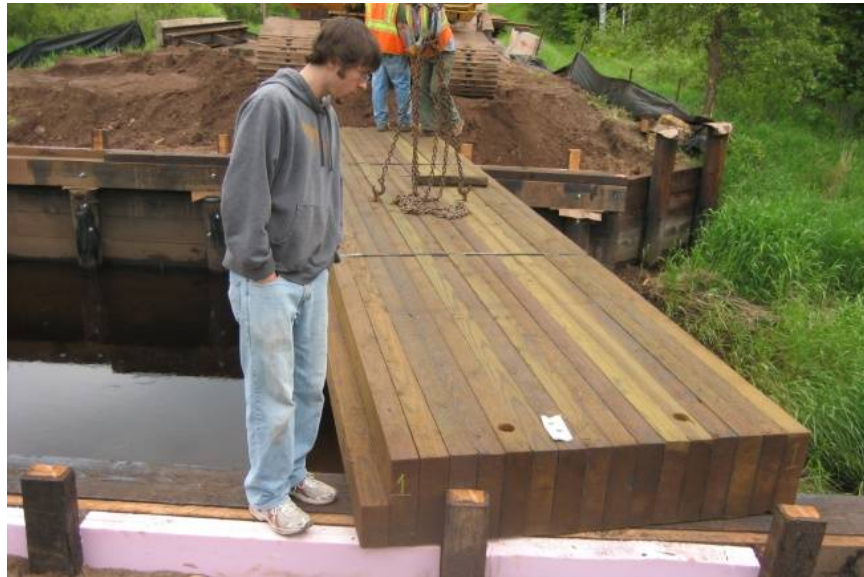
Figure 3.13. Sections were set into place once stays were trimmed and treated.
