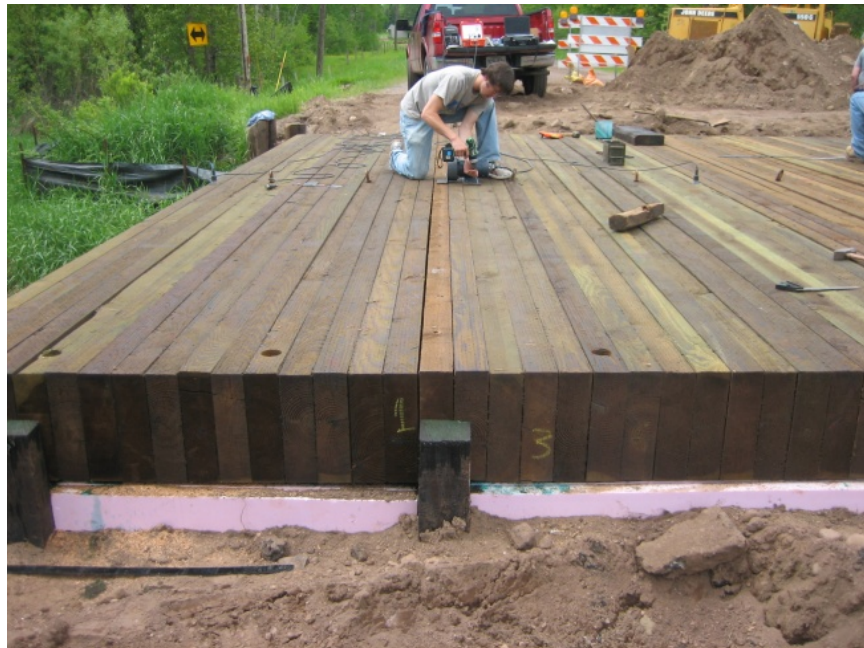
Figure 3.21. Motor being mounted parallel to the laminations in the center of sections 1 and 3.
