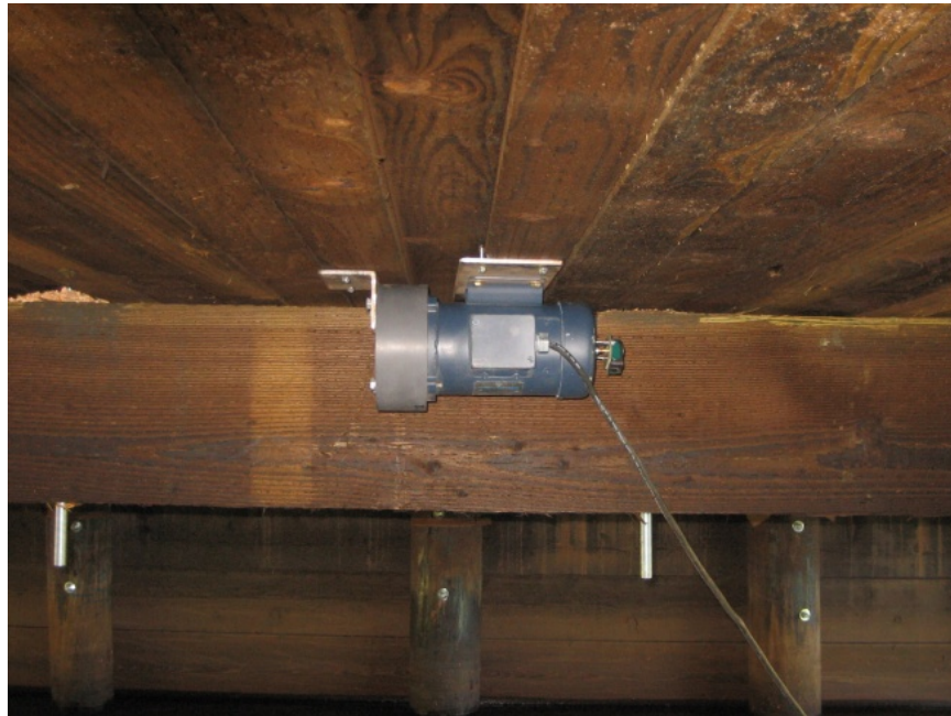
Figure 3.25. Vibration testing with motor mounted below the bridge deck.
