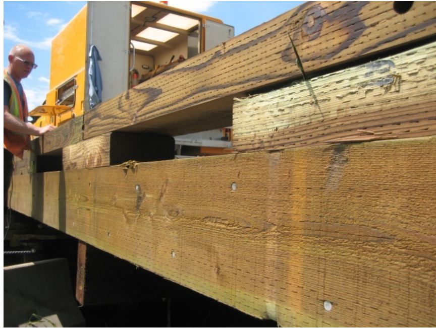
Figure 3.17. Curb being installed on bridge deck.
