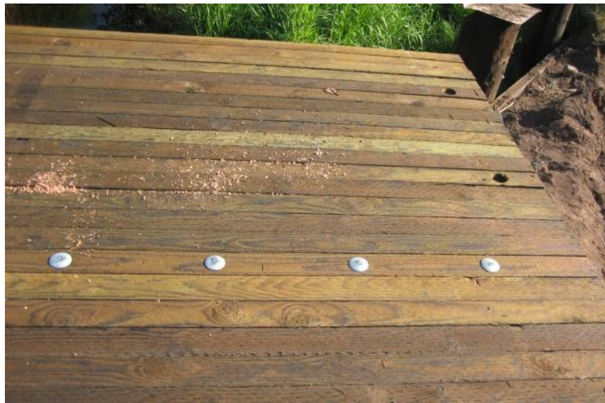
Figure 3.14. Lap joints were pinned together with carriage bolts once sections were set into place.
