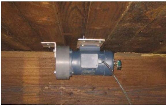
Figure 4.2. General motor attachment on underside of bridge deck for conducting vibration testing.
