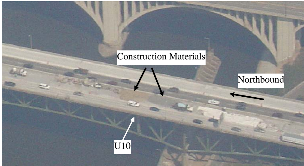
Figure 2.3 Photograph of I-35W Bridge taken prior to collapse on August 1, 2007 (from NTSB 2007).
