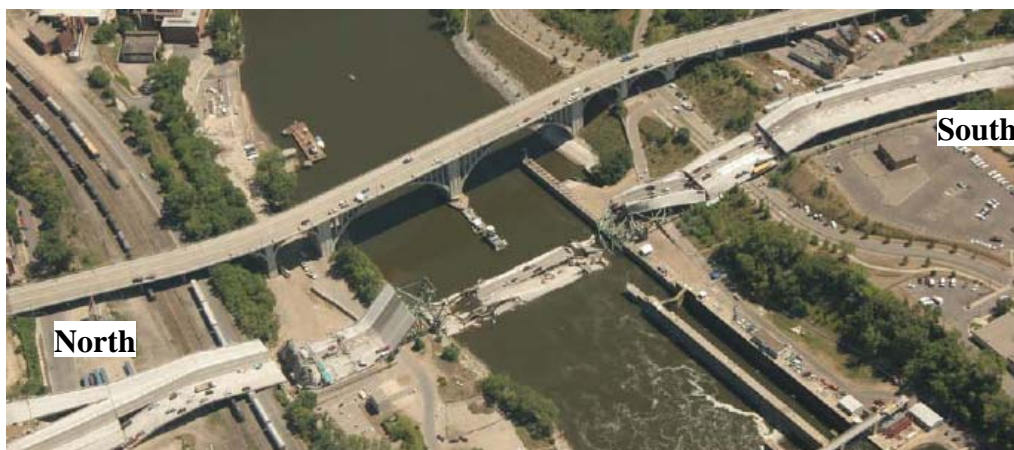
(b) After collapse
