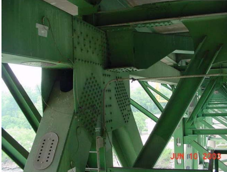
(a) Photograph of U10W before collapse (from NTSB 2008a)
