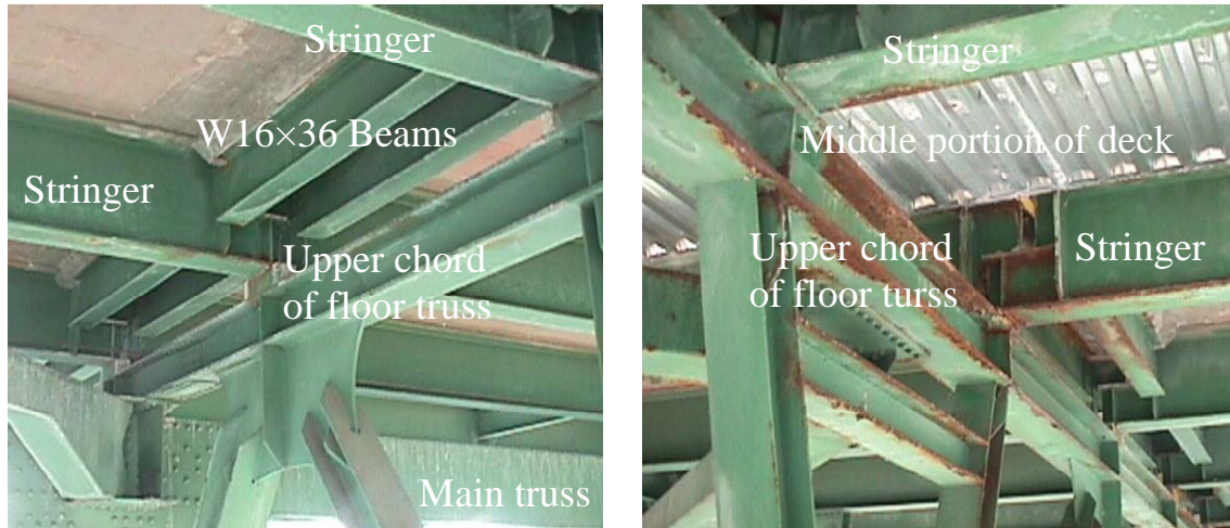
Figure A.13 Photographs of stringer expansions viewed from below (from Prof. Robert Dexter).
