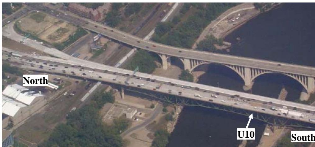
(a) Before collapse
