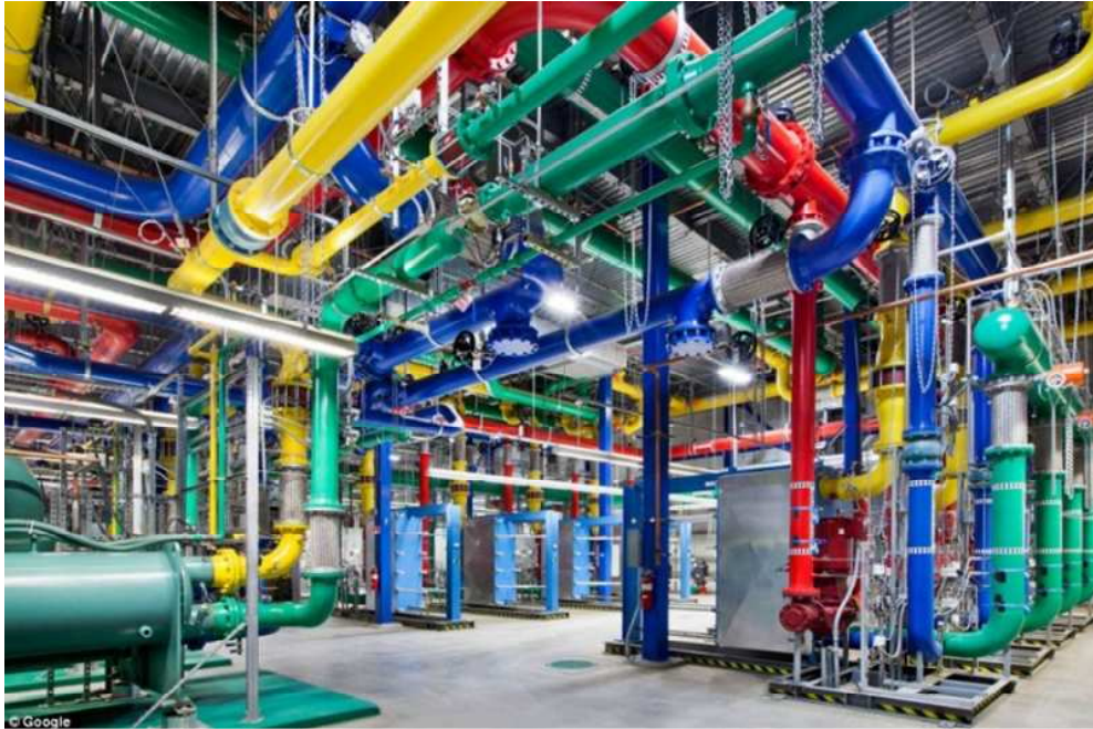
Figure 1.3: Water cooling system in Google's South Carolina center
