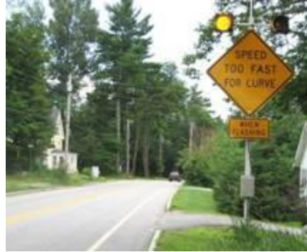
Figure 4.4 Dynamic Curve Speed Warning Sign (with a Flashing Beacon and Radar Detection)
