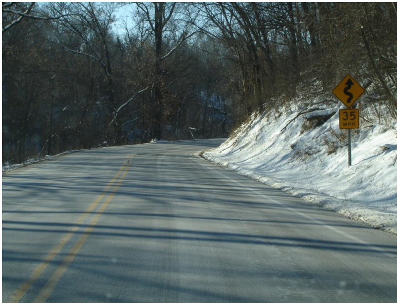
Figure 3.5 Two-Foot Paved Shoulders on TH 60
