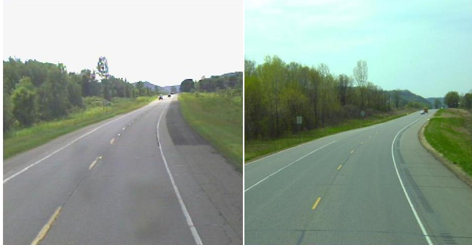
Figure 3.6 On TH 61, Paved Shoulder Through Curve (Before); Paved Shoulder with Rumble Strips Through Curve (After)
