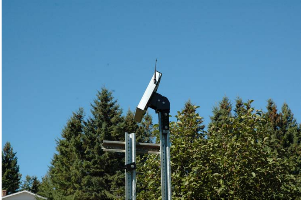
Figure 46: Installed PIR detector.
