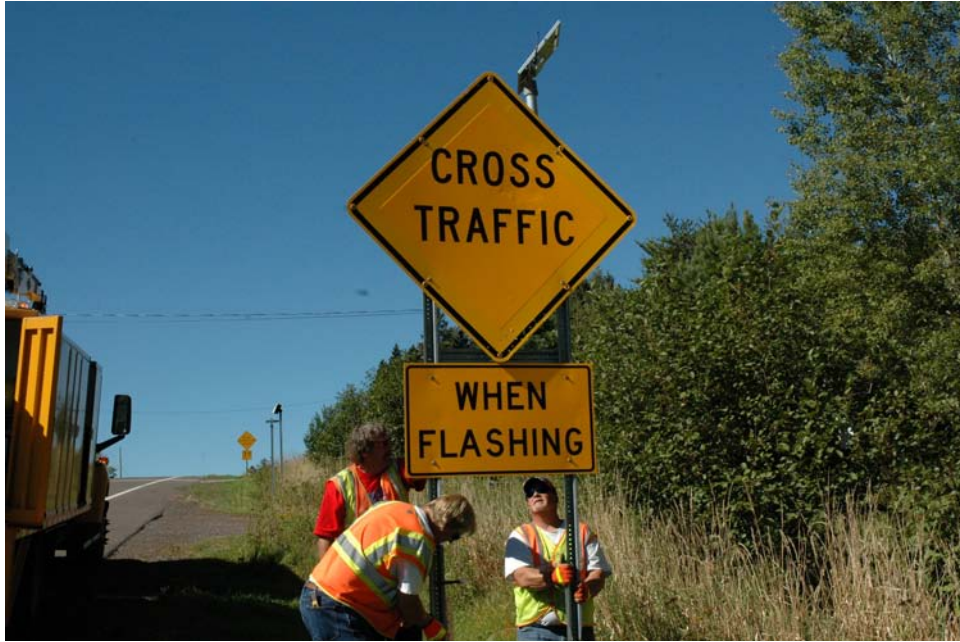
Figure 47: Installed “CROSS TRAFFIC WHEN FLASHING” blinker sign.
