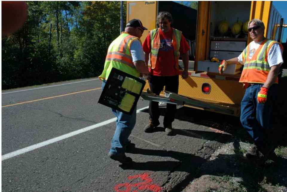
Figure 45: Utility truck holding the PIR detector.
