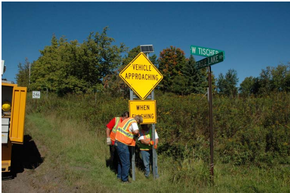
Figure 48: Installed “VEHICLE APPROACHING WHEN FLASHING” blinker sign.
