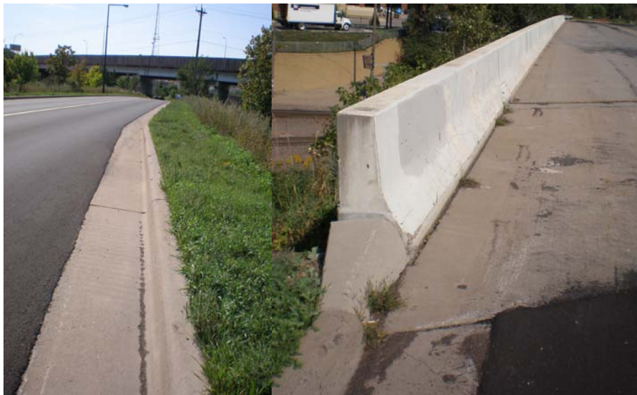
Figure 18. (Left) Regular 'square' curb; (right) Jersey barrier
