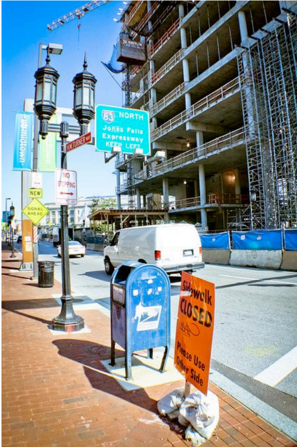
FIGURE 8 . HOTEL UNDER CONSTRUCTION NEAR PENN STATION . PHOTOGRAPH BY AUTHOR
