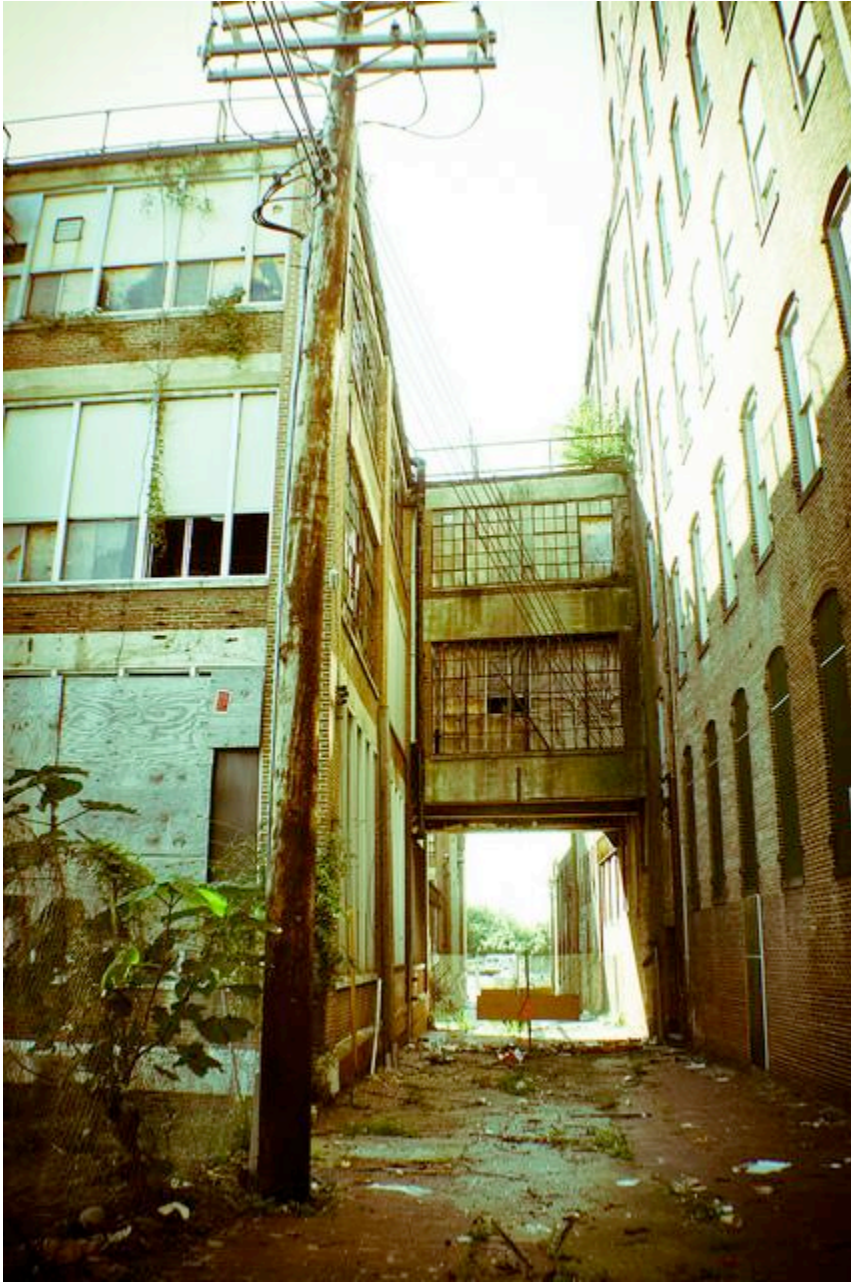
FIGURE 13 . ALLEY BESIDE ABANDONED BUILDING ACROSS FROM THE COPYCAT . PHOTOGRAPH BY AUTHOR
