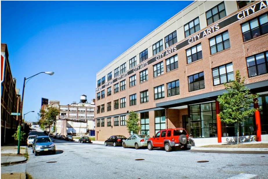
FIGURE 10 . CITY ARTS BUILDING . PHOTOGRAPH BY AUTHOR
