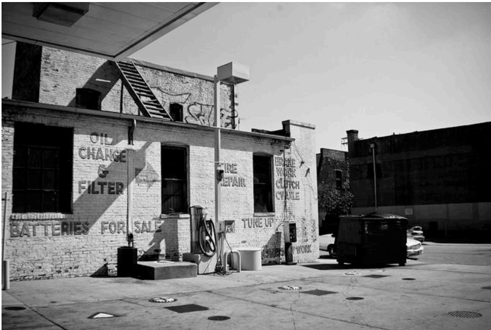
FIGURE 53 . GAS STATION IN STATION NORTH . PHOTOGRAPH BY AUTHOR
