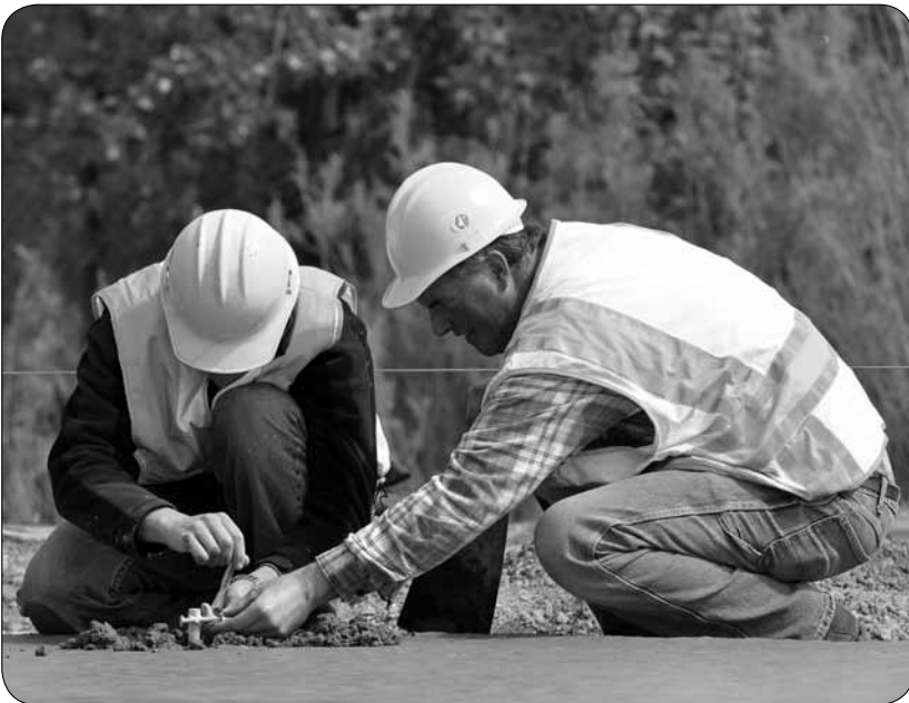
Field experiments at the MnROAD research facility are investigating the use of recycled materials in pavement construction.
