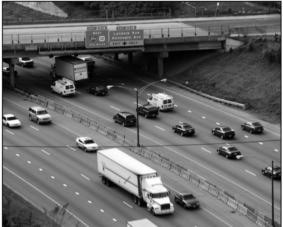
Changes recommended by ITS Institute researchers have improved traffic flow and safety at this stretch of I-94 in Minneapolis.
