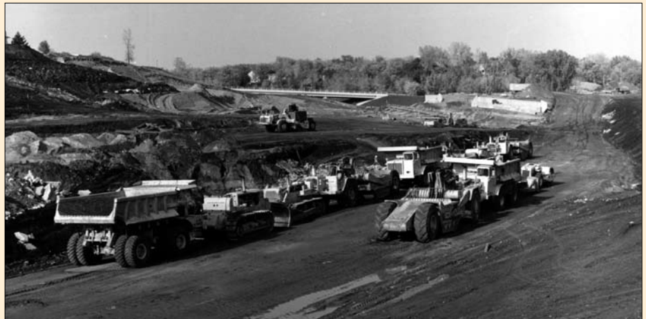
I-35E construction during the 1960s in St. Paul, Minnesota
