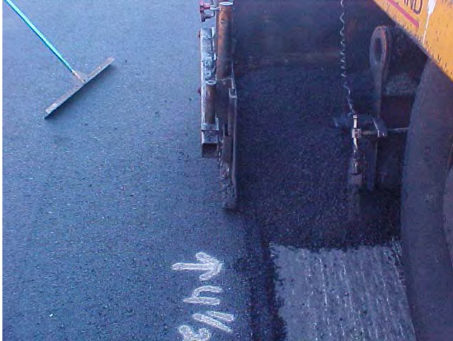
Figure 5-13: Proper overlap of hot mat onto cold mat (Benson and Scherocman 2006).
