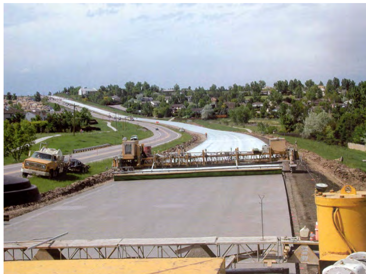
Figure 5-1: Curing of concrete pavements is critical; water cure eliminates built-in temperature gradients, high zero-stress temperature, and excessive shrinkage.
