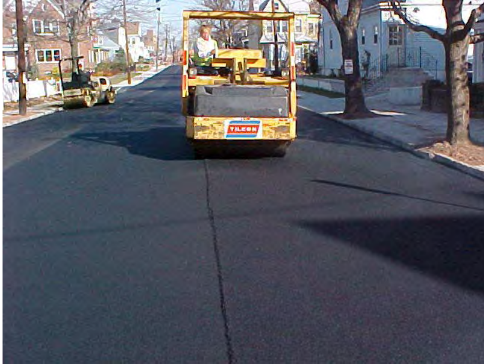
Figure 5-14: Rolling of hot mat for joint compaction (Benson and Scherocman 2006).
