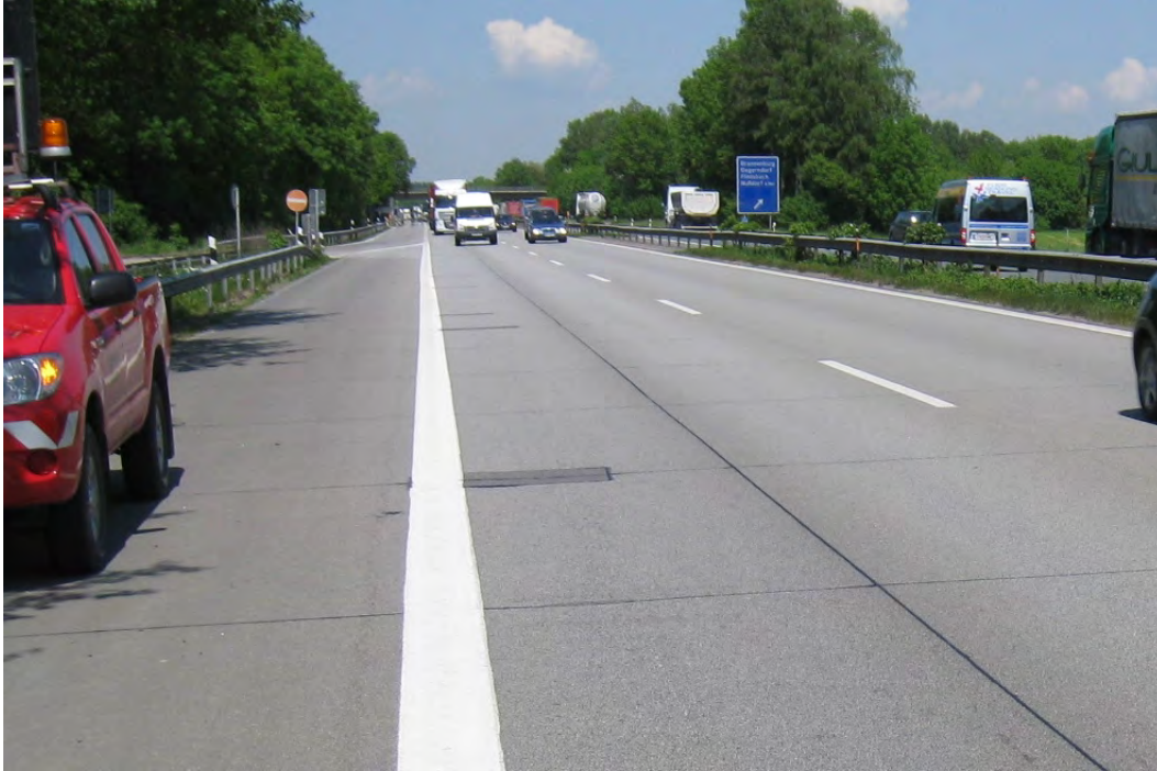
Figure 5-17: SMA over PCC along A93 in Germany, rectangular patch repair visible next to red traffic diversion truck (Rao SHRP 2010).
