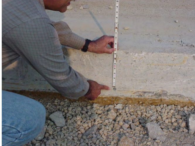
Figure 5-3: Tie bar placement is important and should be measured every day.
