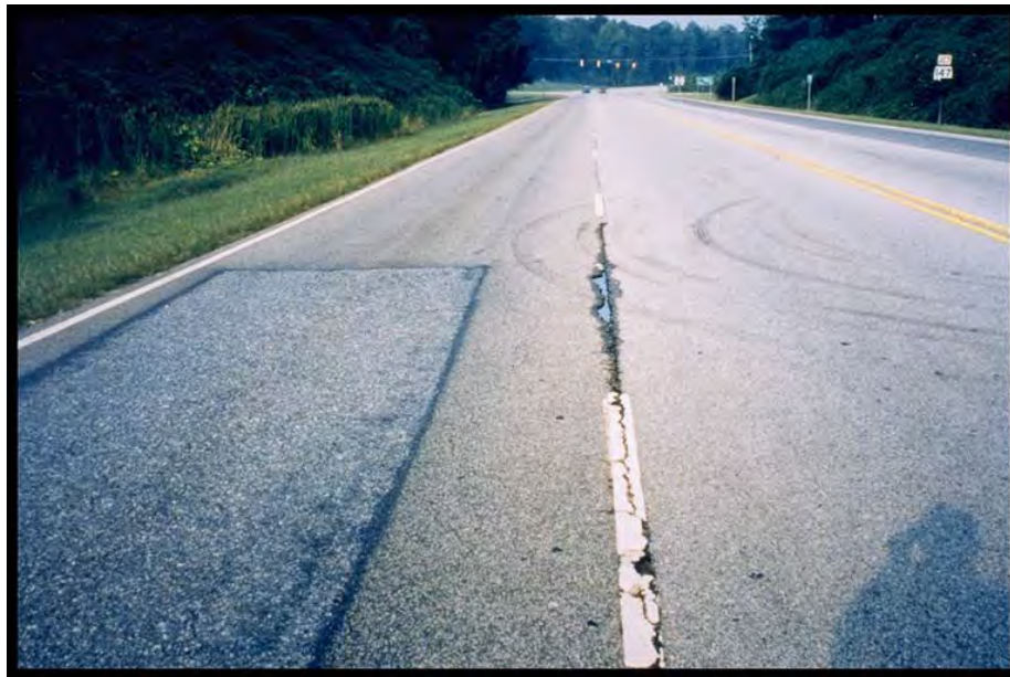
Figure 5-11: Raveled longitudinal joint (Brown, 2006).
