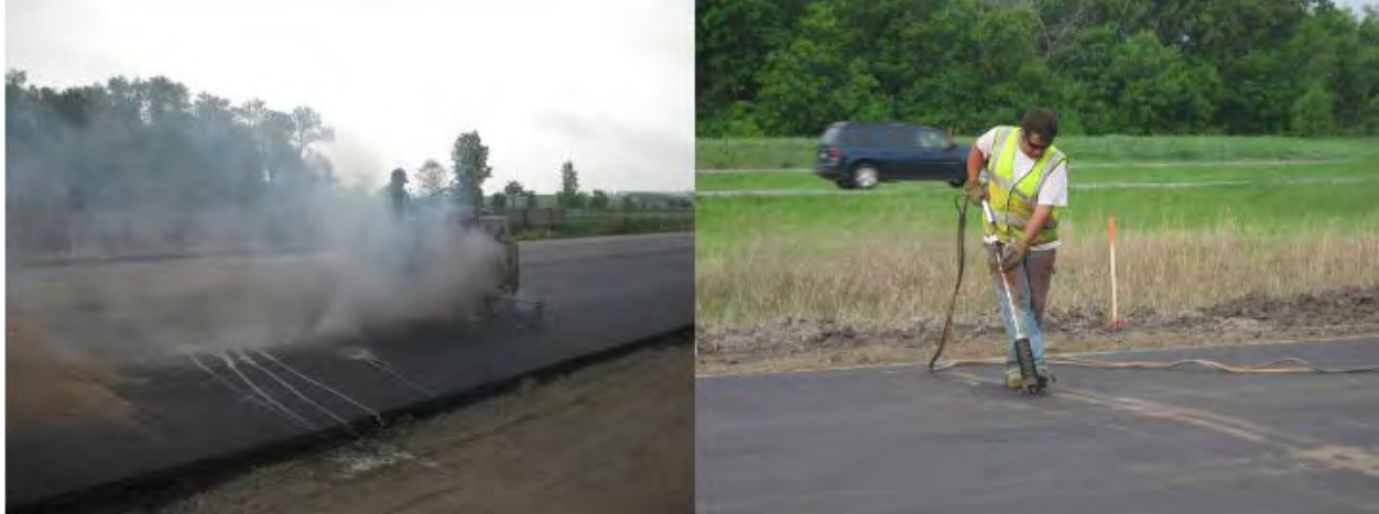
Figure 5-15: Sawing joints in the AC layer which correspond to the joints in the underlying PCC layer (left) and sealing the newly sawn joints (from Rao et al 2011).
