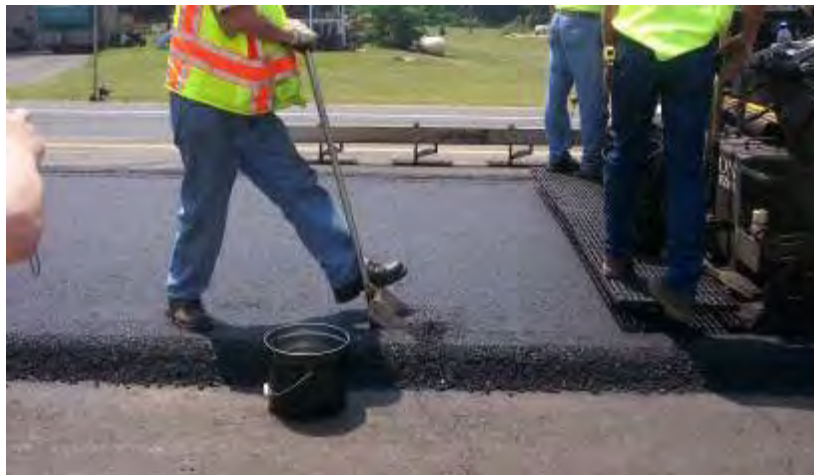
Figure 5-20: Shoveling material from above plates.
