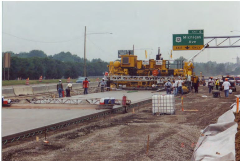
Figure 5-4: Quality construction is critical and contractor pay incentives are very helpful.
