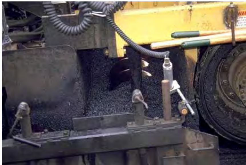
Figure 5-9: HMA head in auger (Mahoney, Pavement interactive.com).
