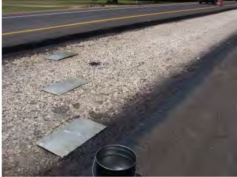
Figure 5-19: Plates randomly placed under HMA mat.
