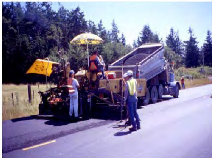
Figure 5-8: End dump of HMA into paver hopper (Mahoney, Pavement Interactive.com).
