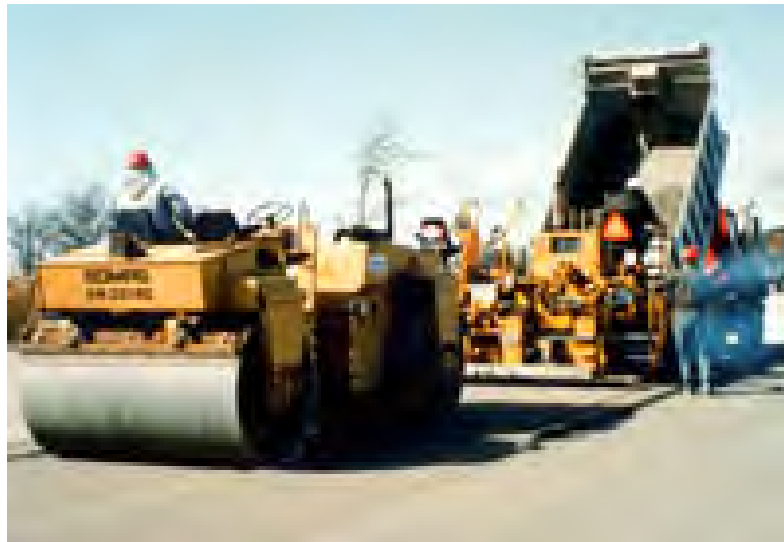
Figure 5-6: Typical RCC paving operation: dump truck unloads mix into an asphalt paver, a roller follows close behind to ensure adequate compaction (from Portland Cement Association, 2012).
