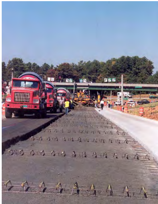
Figure 5-2: Dowels can be placed within acceptable tolerances, field measurement every day is critical.
