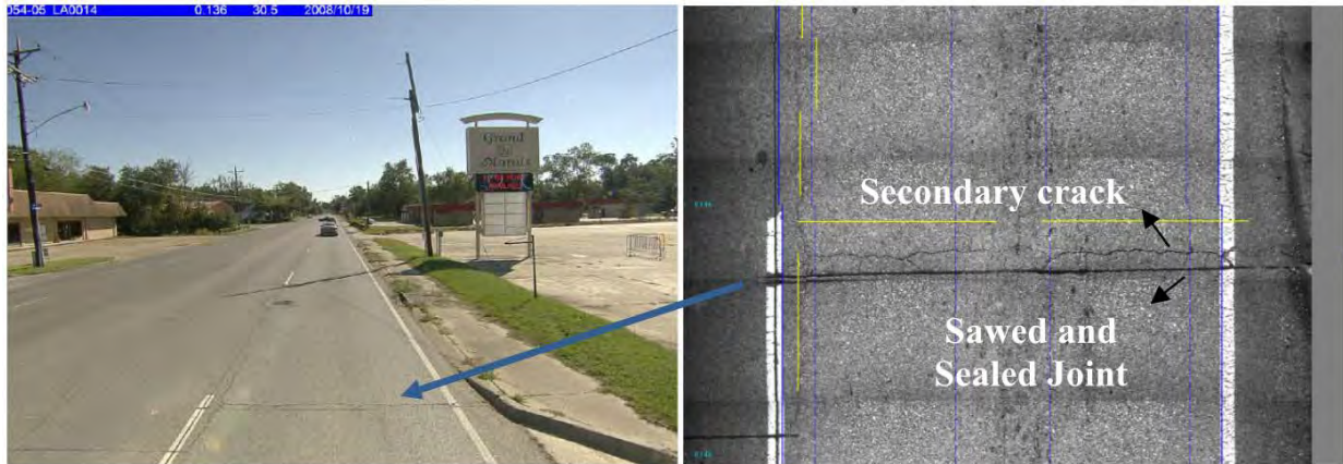
Figure 5-16: Illinois tollway saw-and-seal (Elsefi 2011).
