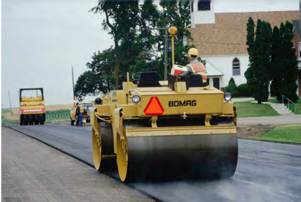
Figure 5-12: Proper rolling of free edge (Benson and Scherocman 2006).
