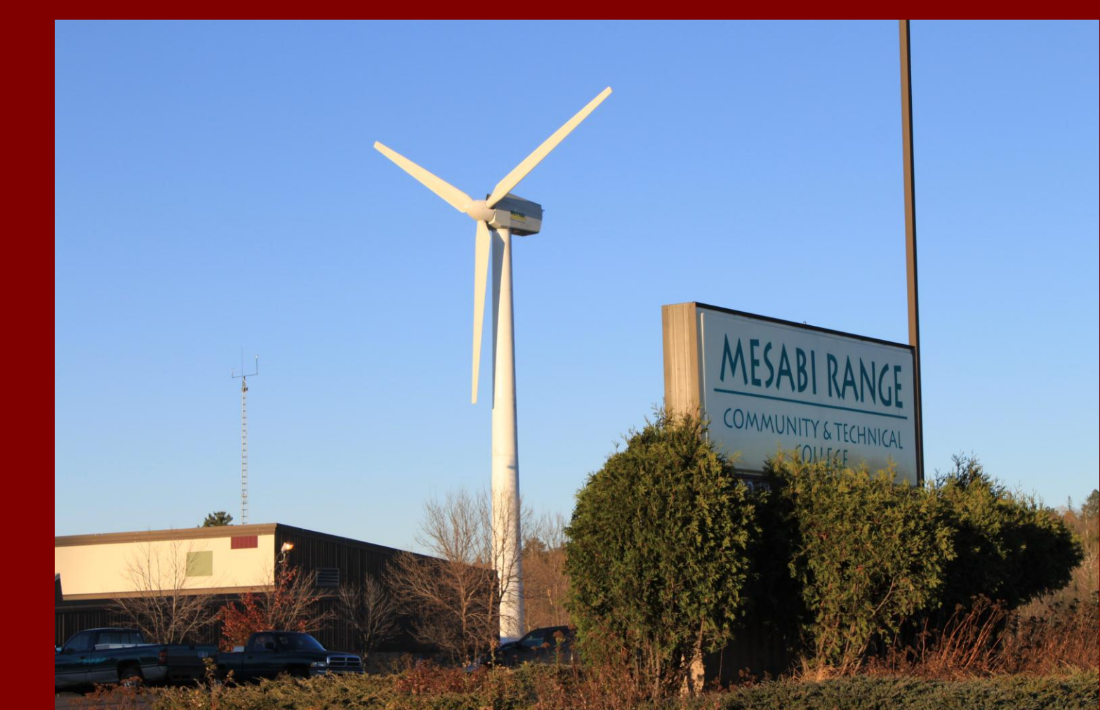
Figure 7: This is a picture of the Vestas V27 turbine at Mesabi Range Community and Technical College [5].
