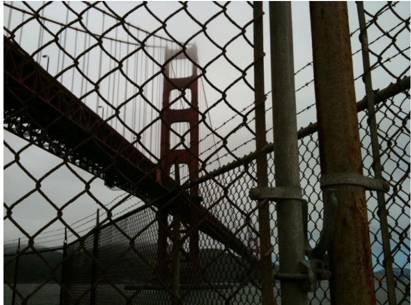
Figure 2.1 Contemporary View of Fort Point
