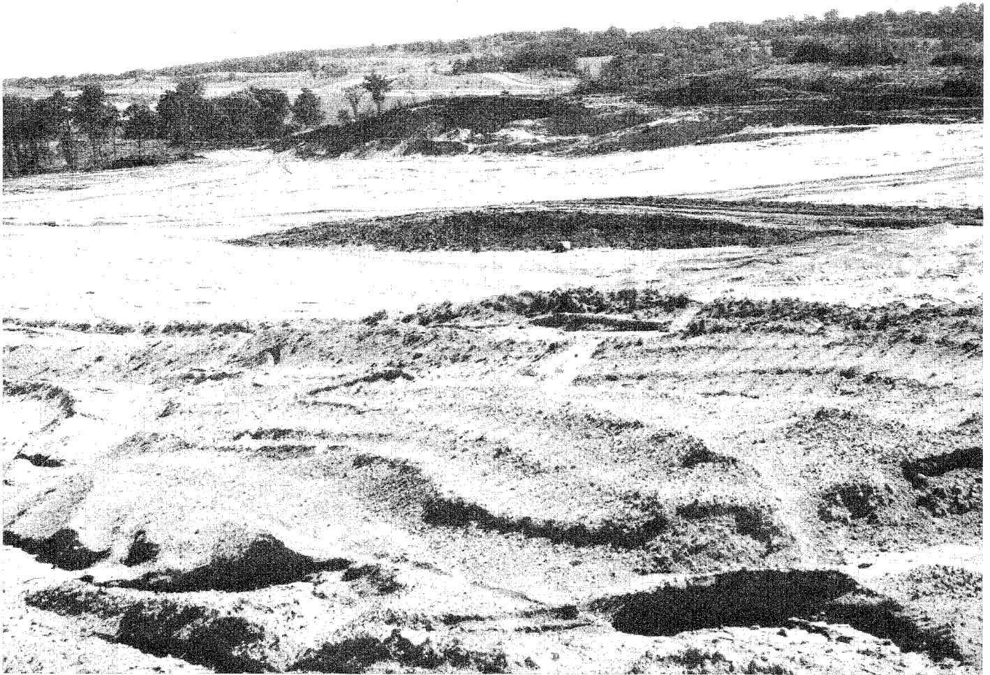
Site preparation for building construction often subjects the land to a period of increased erosion.
