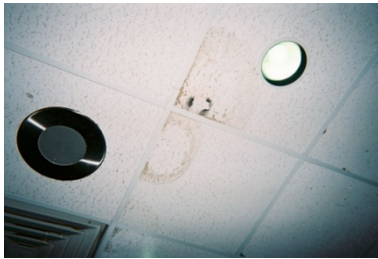
Figure 15: Stained ceiling tiles
