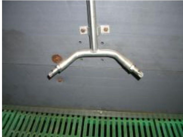
Figure 2: Solid mounted nipple drinker (The Pig Site, 2010). Note that water not consumed by pigs falls through the slatted floor into the manure slurry storage.
