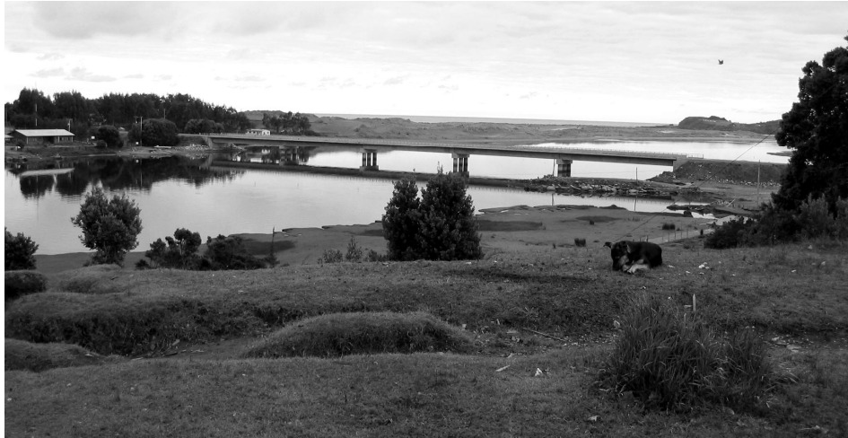
Figure 1.1: Bridge over the Chaihuín River. The view here is from the northern bank. The headquarters of the Valdivian Coastal Reserve are visible to the left, at the far end of the bridge. The estuary can be seen in the upper right of the photo and beyond it the Pacific Ocean.
