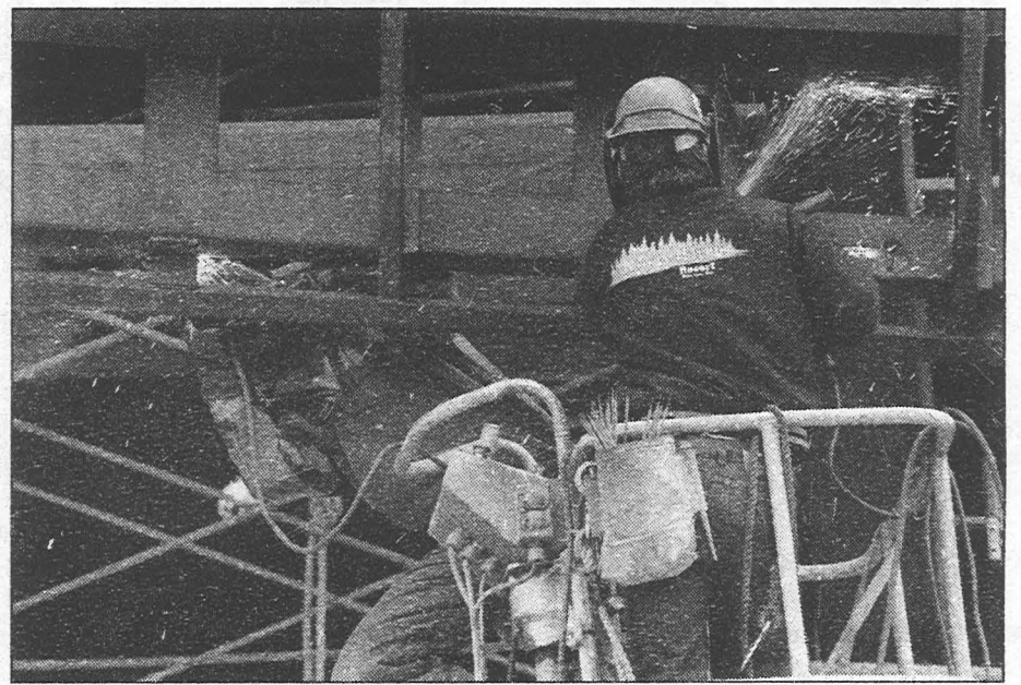
Workers weld supports on the new University art gallery. An initial $3 million challenge pledge from former student Frederick R. Weisman enabled construction. The museum, designed by internationally renowned architect Frank O. Gehry, is scheduled for completion in fall 1993. (Photo by Dilip Vishwanat)
