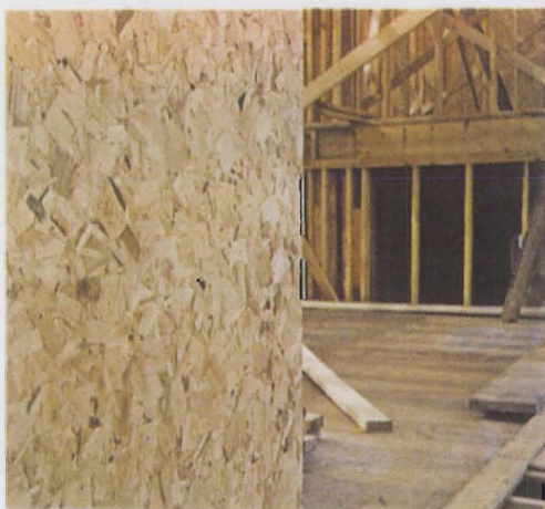
Waferboard offers promise as wall sheathing in residential construction (photo by Roland Gertjejansen).
