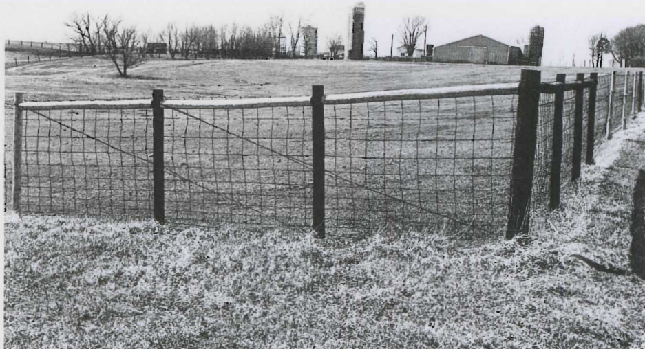
Development of the multiple-post "Rosemount fence corner" has given farm and right-of-way fences a sturdy, economical foundation.
