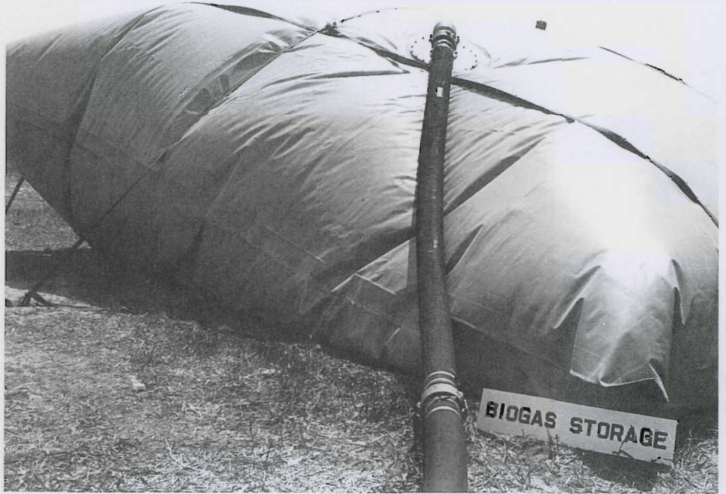
Manure from Verlo Larson's swine finishing operation produces 800 cubic feet per day of methane (bio-gas) via an anaerobic digester system. When the system is perfected, the stored bio-gas could be used to operate a motor generator system to produce part of his electrical needs (photo by Mel Kiser).
