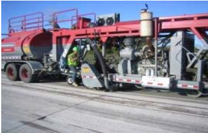
Diamond Grinding Process and Surface Created
