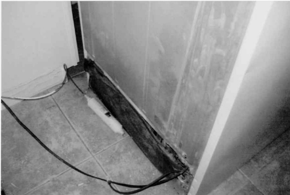
Figure 21: Photograph of a return where the filter was plumbed with copper tubing and was unsupported. As the tubing stiffens over time due to cold work the bending forces produced will continue to increase.
