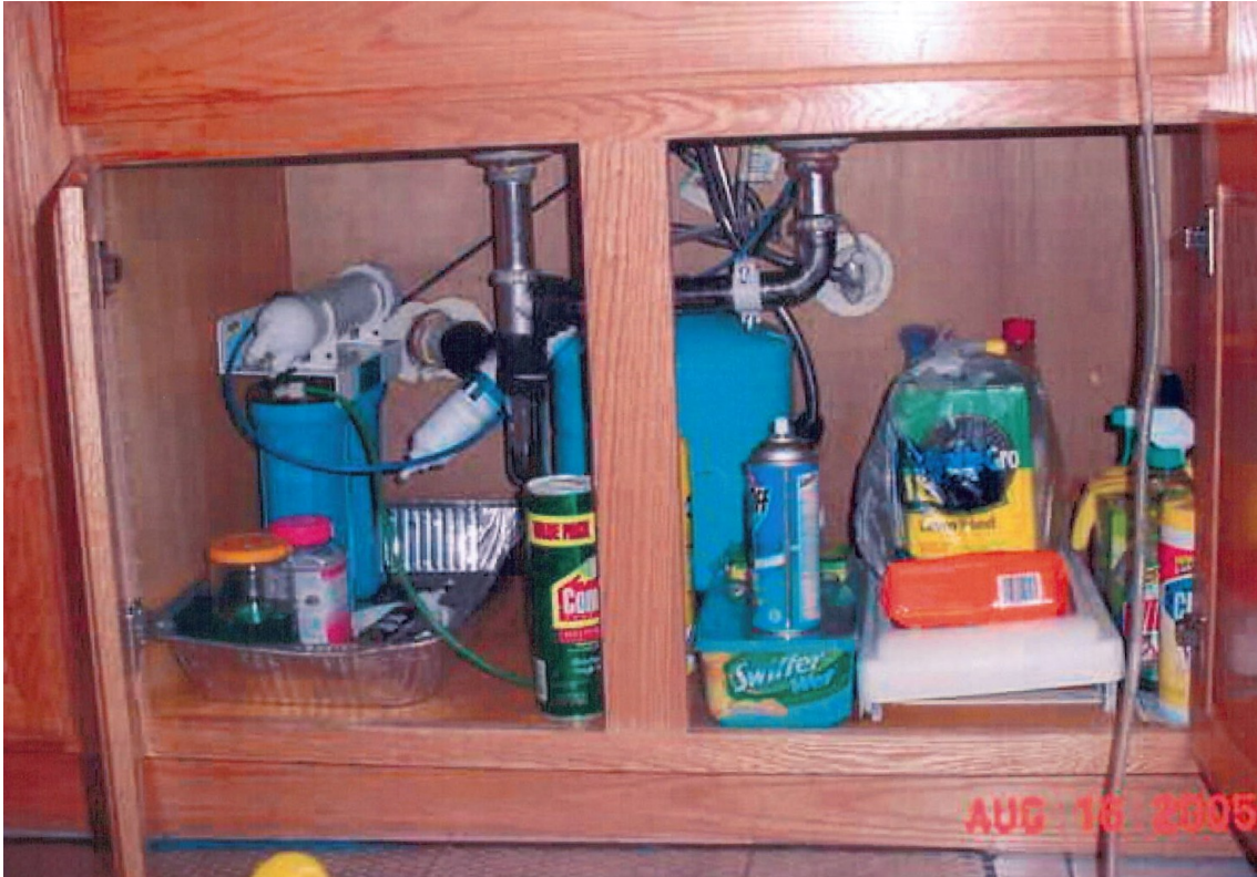
Figure 23: Photo of a filter installation under a sink. The kind of tubing used is unknown, but this filter was plumbed with hot rather than cold water, and was an inlet filter to an "instant" water heater.
