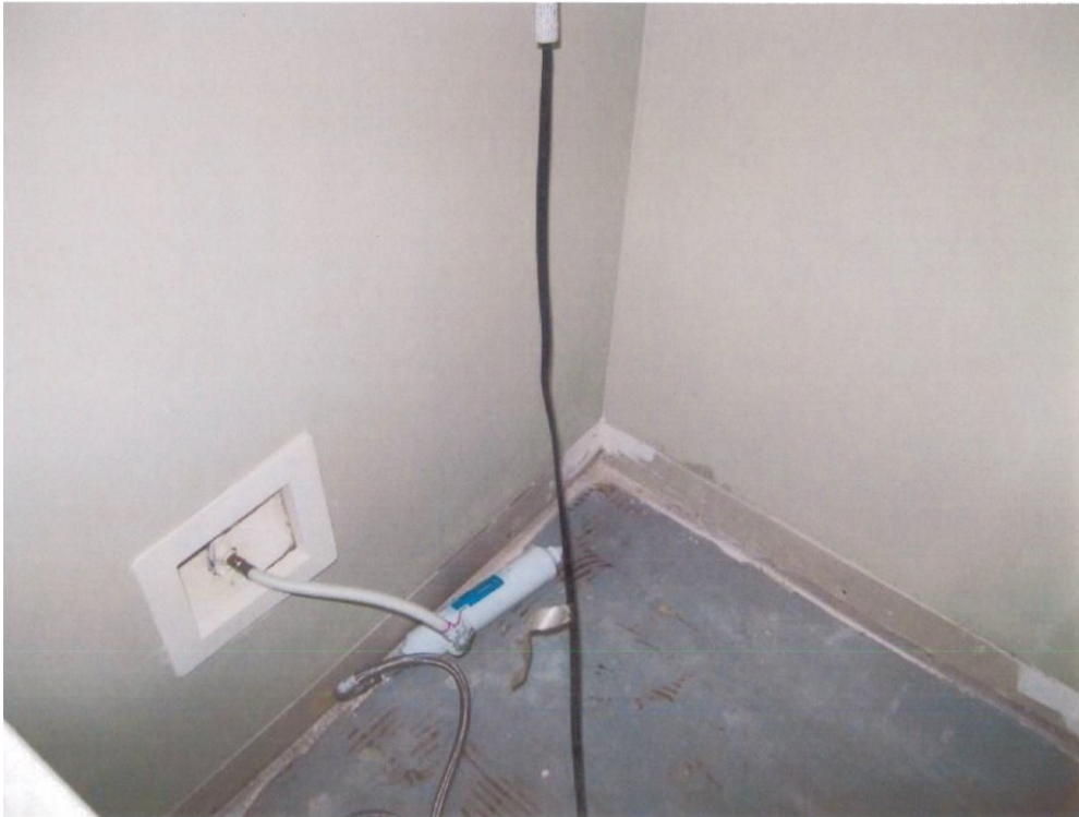
Figure 22: Photo of a filter installation where braided tubing was used and the filter appears to be unsupported.
