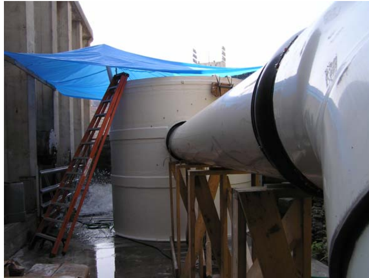
Figure 2.2. The 24-inch influent pipe and a Modified Model 3 ecoStorm on the Turbine level of SAFL.
