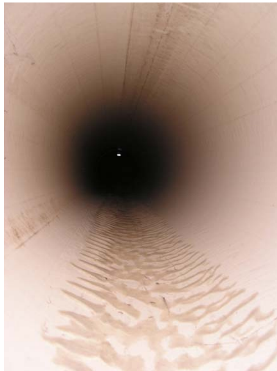
Figure 4.1. Deposition of the solids in the influent pipe under low flow conditions.
