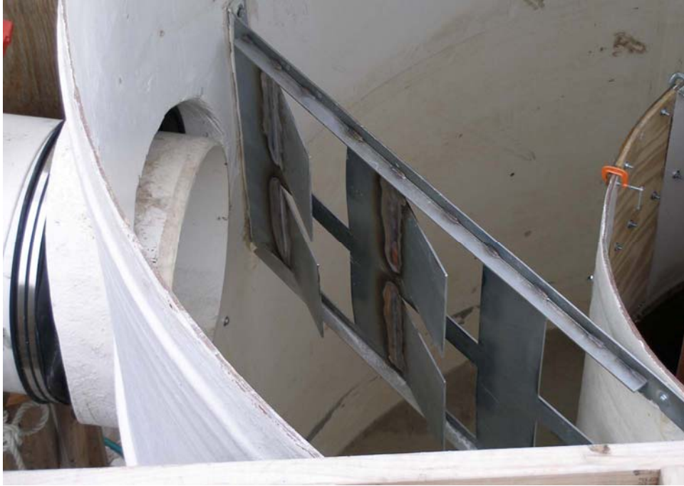
Figure 1.3. The diversion plate inside the manhole at the outlet of the influent pipe.
