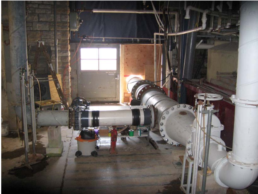
Figure 2.1. The 12-inch supply pipes, the 12 to 24-inch expansion and the control valves of the test stand.
