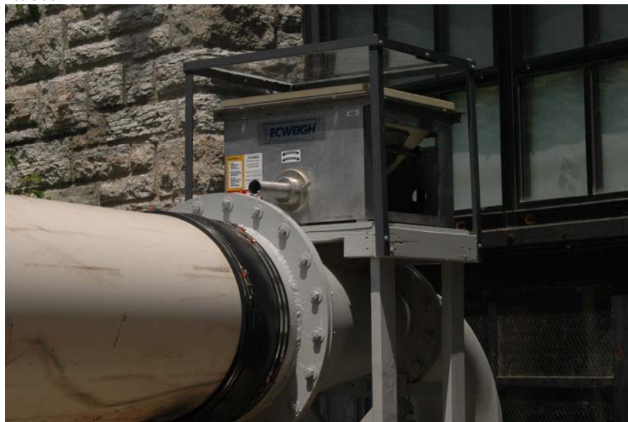
Figure 2.4. The sediment feeder at the upstream end of the 24-inch influent pipe.
