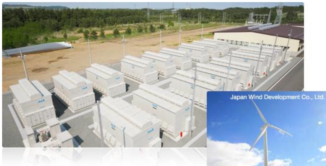
Figure 43: 34MW NaS Installation at Rokkasho Wind Farm, Japan [61]
