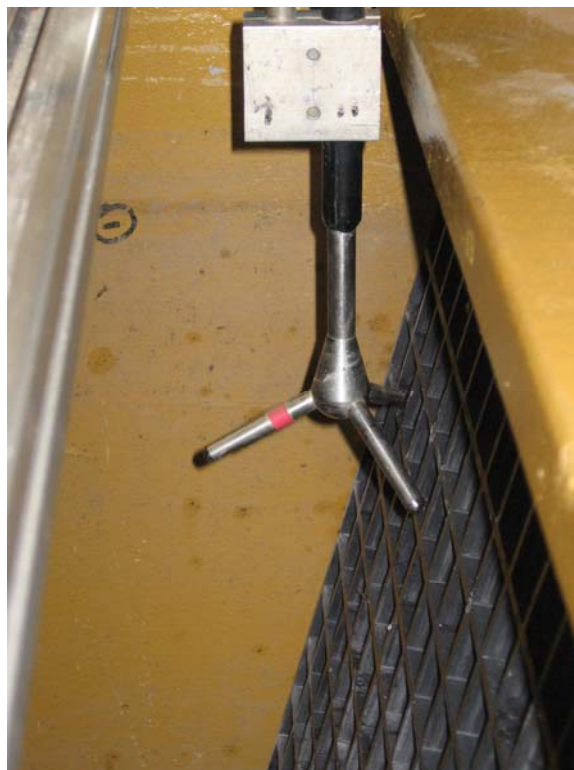
Figure 9. The three-dimensional Acoustic Doppler Velocimeter (ADV) to measure approach velocity approximately one inch upstream of the trash rack.
