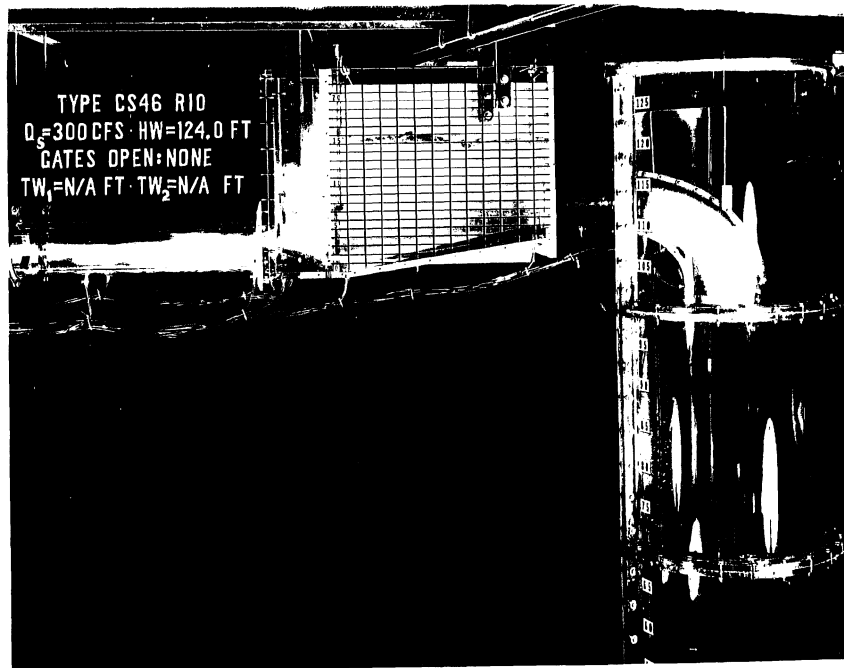
Photo 54 - Type CS46 R10 control structure, Q_s = 300 cfs, H.W. = 124.0 ft, no gates open, T.W.1 = N/A, T.W.2 = N/A. The bifurcation structure.
