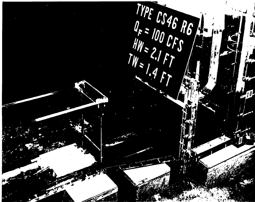
Photo 25 - Type CS46 R6 control structure, Q_F = 100 cfs, H.W. = 2.1 ft, T.W. = 1.4 ft. The pinch area.
