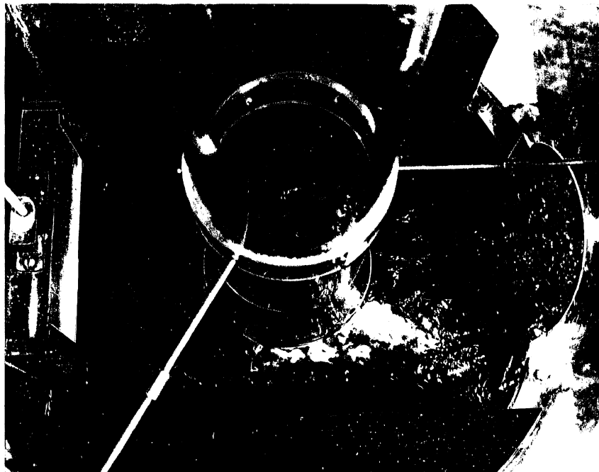
Photo 20 - Type CS46 R4 control structure, Q_F = 100 cfs, H.W. = 2.1 ft, T.W. = 1.5 ft. The surge shaft invert and siphon riser.
