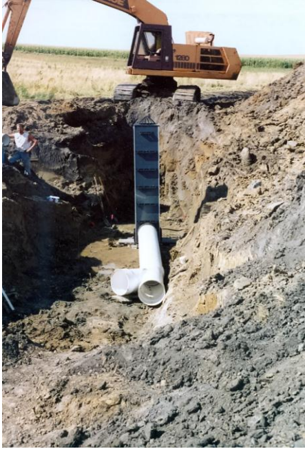
Figure 1.2 Outlet structure installation.
