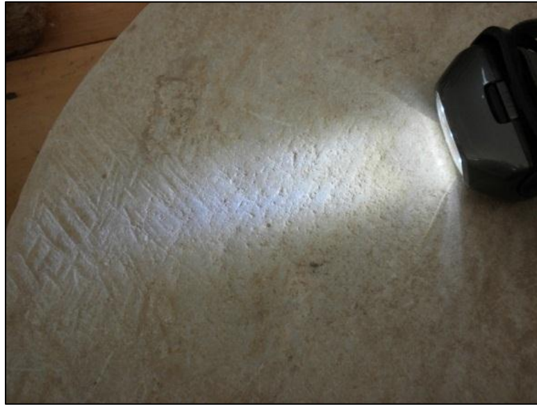
Figure 137. Wear pattern on the surface of column base A 8 (photo by author).
