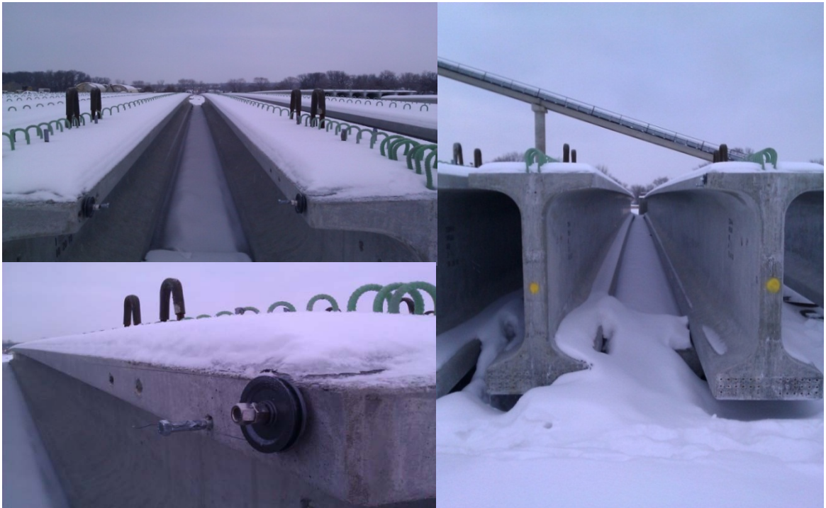
Figure 7-7. Winter environment for girders at Plant A
