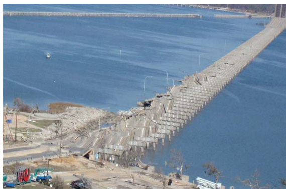
(c) Collapsed bridge.
