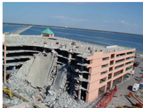
(b) Damaged parking garage.
