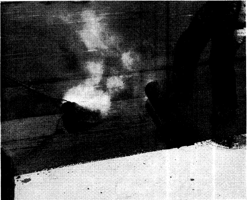
Solid Mopping of Roofing Felts
