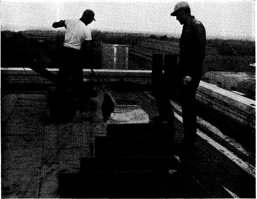
Solid Mopping of Roof Decks
