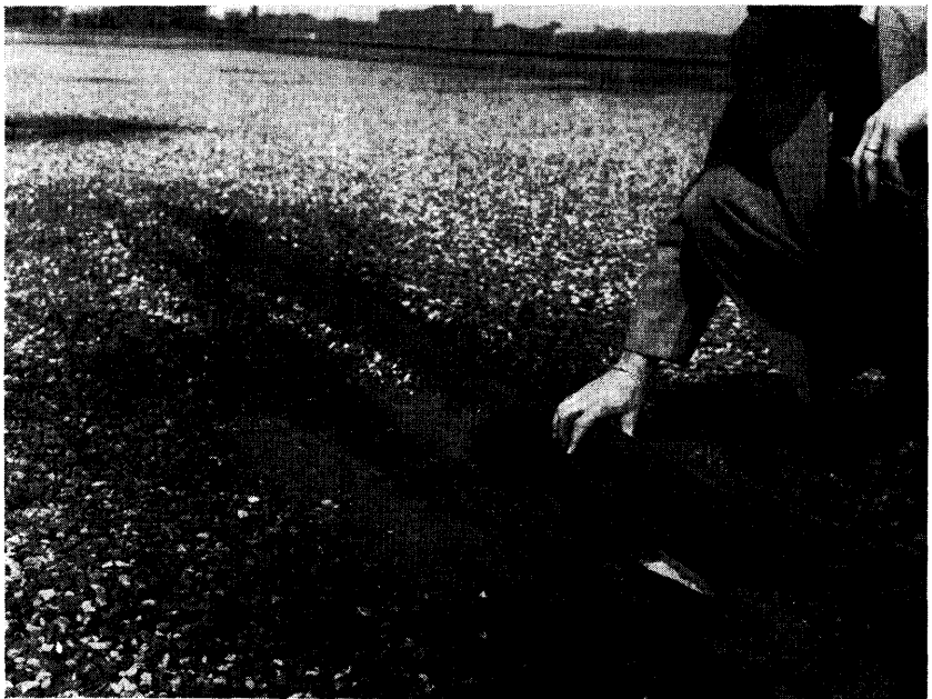
Structural Roof Blisters Showing Expansion of Felts
