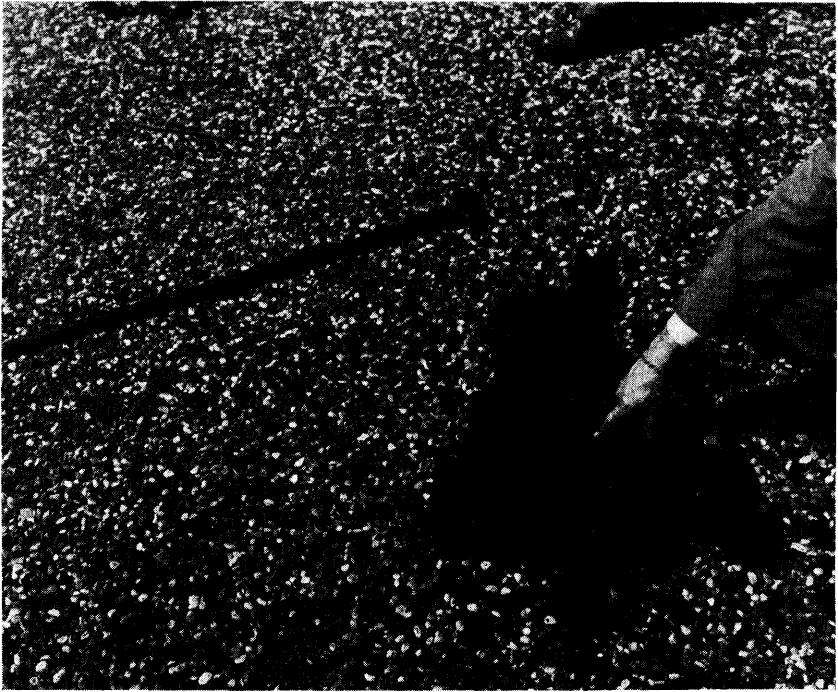
Structural Roof Blisters with Water Between Felts
