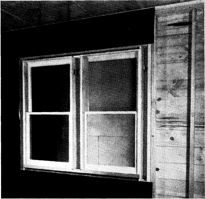
FIGURE 14. VIEW OF INTERIOR SURFACES OF WALL BEFORE LATH AND PLASTER WERE APPLIED SHOWING INSTALLATION OF CONTINUOUS BARRIER, WALL WITHOUT INSULATION, AND DOUBLE WINDOW WITH INTERIOR TRIM REMOVED.
