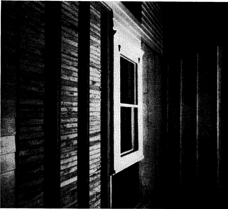
FIGURE 10. VIEW OF EXTERIOR WALL WITH OUTER WALL SECTION REMOVED SHOWING DIFFERENT TYPES OF INSULATION, WINDOW INSTALLATION, AND OUTER WALL SECTION WITH REMOVABLE SHEATHING PANELS.
