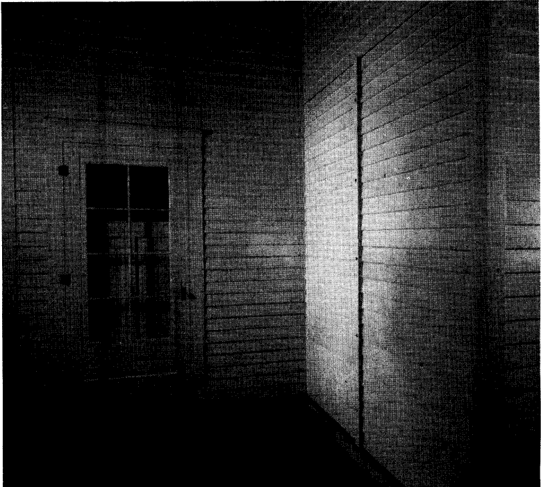
FIGURE 9. VIEW OF ENTRANCE TO BUNGALOW SHOWING THE EXTERIOR WALLS COMPLETELY ASSEMBLED.
