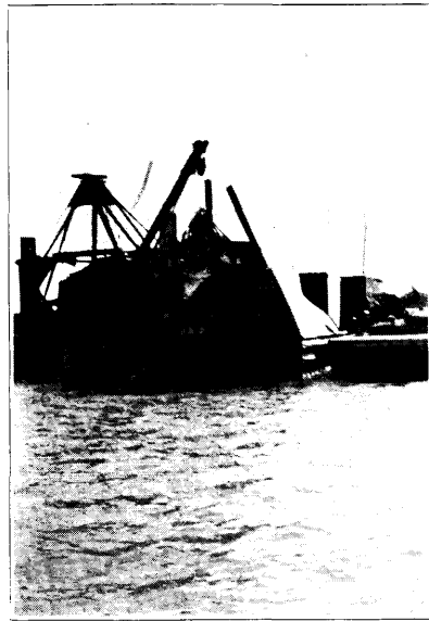
FIGURE 4. LOADING MARL IN SCOWS AT AETNA PORTLAND CEMENT COMPANY
