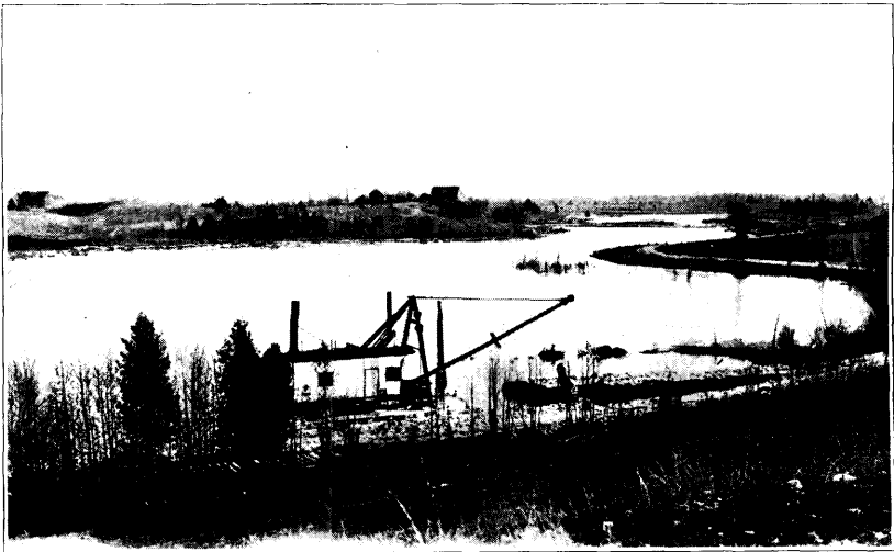
FIGURE 2. MARL LAKES OF HANOVER CEMENT COMPANY SHOWING DREDGE
