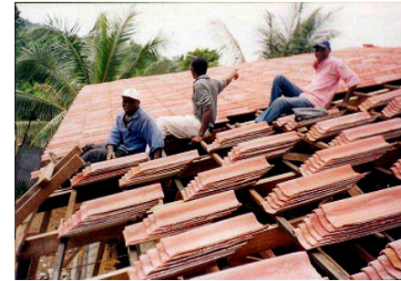
6.1 Micro Concrete Tiles (MCR) Roofing alternative that reduces cost and uses local resources.
