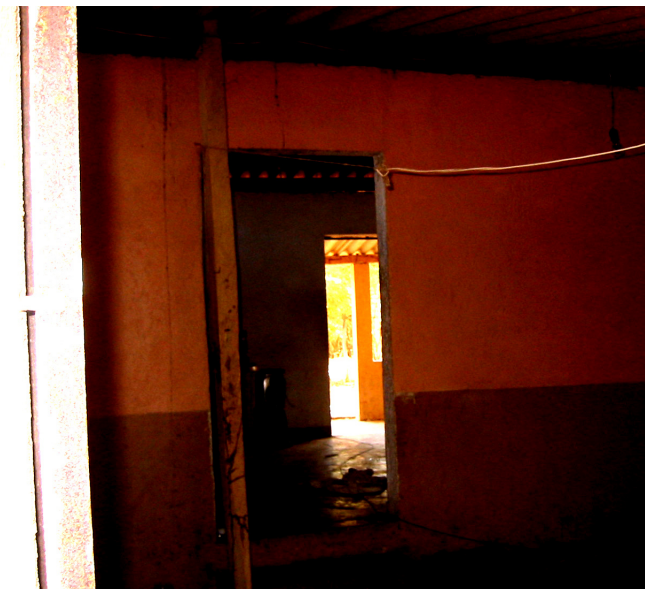
1.2 Existing House hot and segmented living spaces
