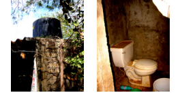
potable water used for toilet
