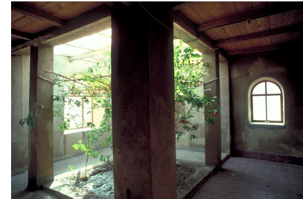
4.1 Hassan Fathy: Stopplaere House Fathy incorporated dense brick walls and traditional courtyard forms to provide passive cooling.
