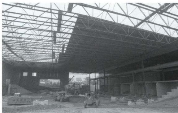
Right: The Ridder Arena and Tennis Facility construction site on September 18, 2001.
