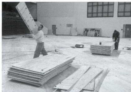
Left: Facilities staff work to dry and clean the Pavilion floor after the warped boards were stripped and trashed.
