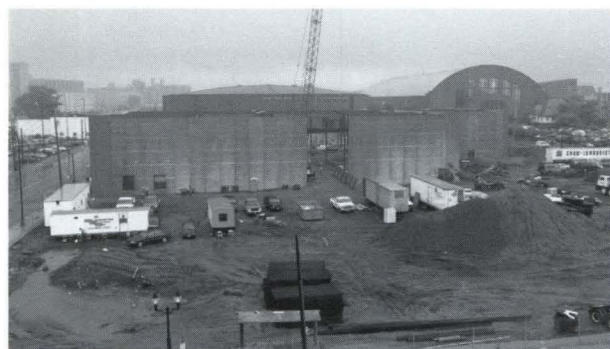
Left: The Ridder Arena and Tennis Facility construction site on July 19, 2001.
