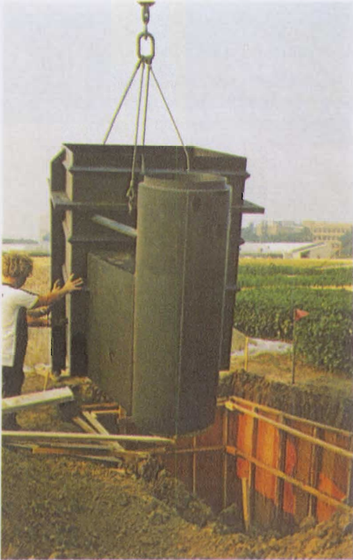
This "box" or weighing lysimeter being lowered into the soil will help tell when to irrigate and how plants consume water. A scale is attached to the apparatus to measure weight differences due to water gain or loss by the plants and soil (photo by Don Baker).
