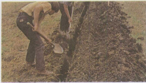
Workers backfill a UM Nutrient Movement Plot.
