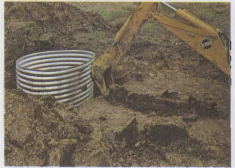
A culvert to be used as a water collection pit is placed in a Nutrient Movement Plot.
