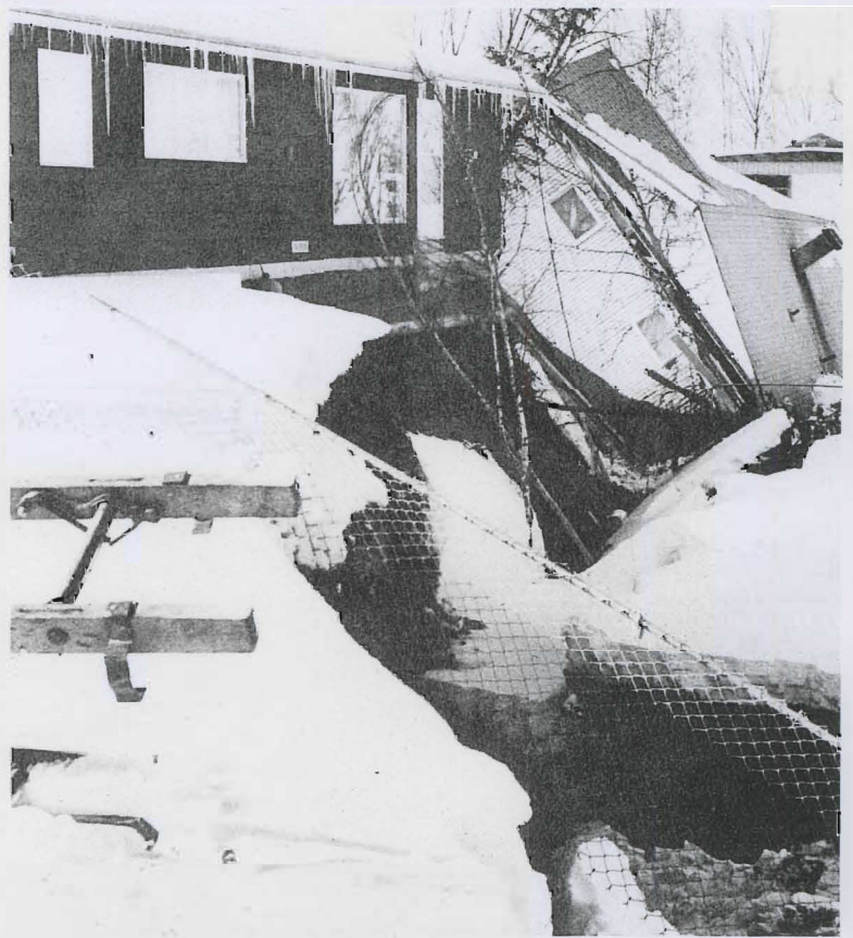
The 1964 Alaskan earthquake toppled this home from its foundation but the wood house held its shape and helped protect the lives of its occupants.
