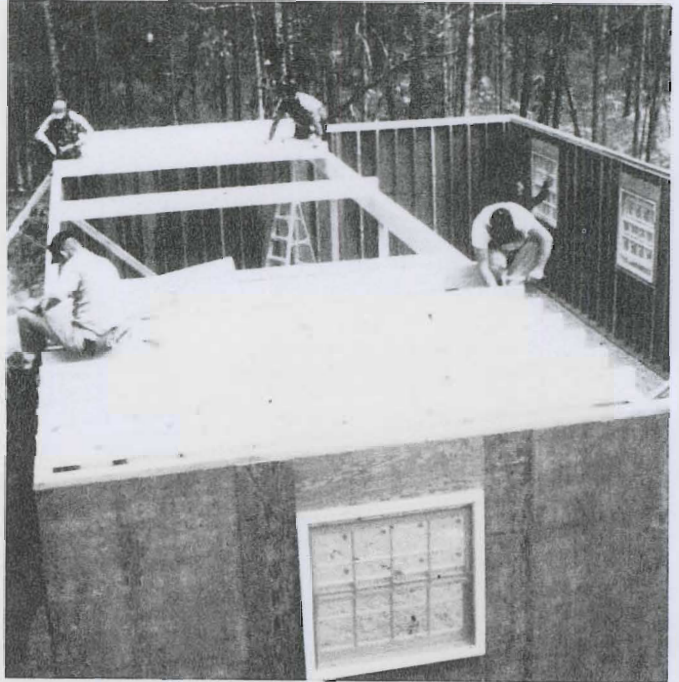
All weather wood foundations eliminate the need for concrete in homes. Pressure-treated wood footing plates rest on a 4-inch or thicker bed of gravel.
