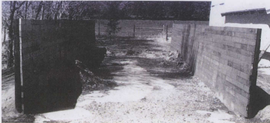
Horizontal silo made of treated posts and lumber.
