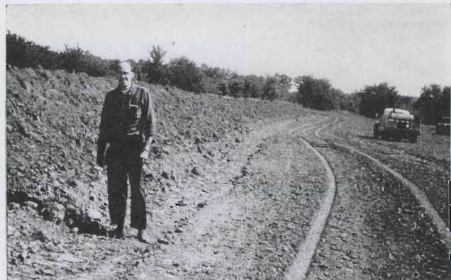
Figure 3. Lower side of finished push-up level terrace on an 8-percent slope, replacing old-style terrace. Note greatly reduced slope between terraces.
