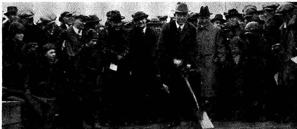
President Coffman turns the first spadeful of dirt, initiating the construction of the Memorial Stadium
