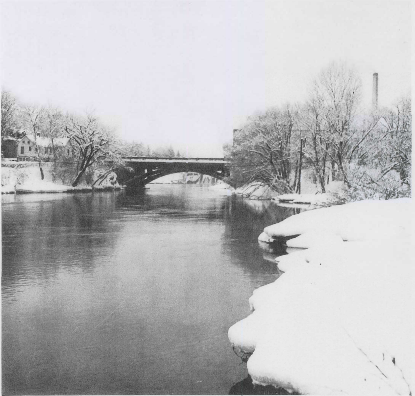
A cold day below Prairie River dam, Grand Rapids.
